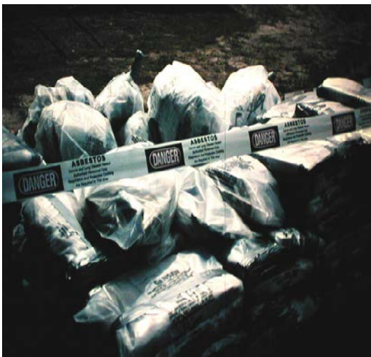
Waste asbestos must be properly bagged, labeled, and disposed of.
