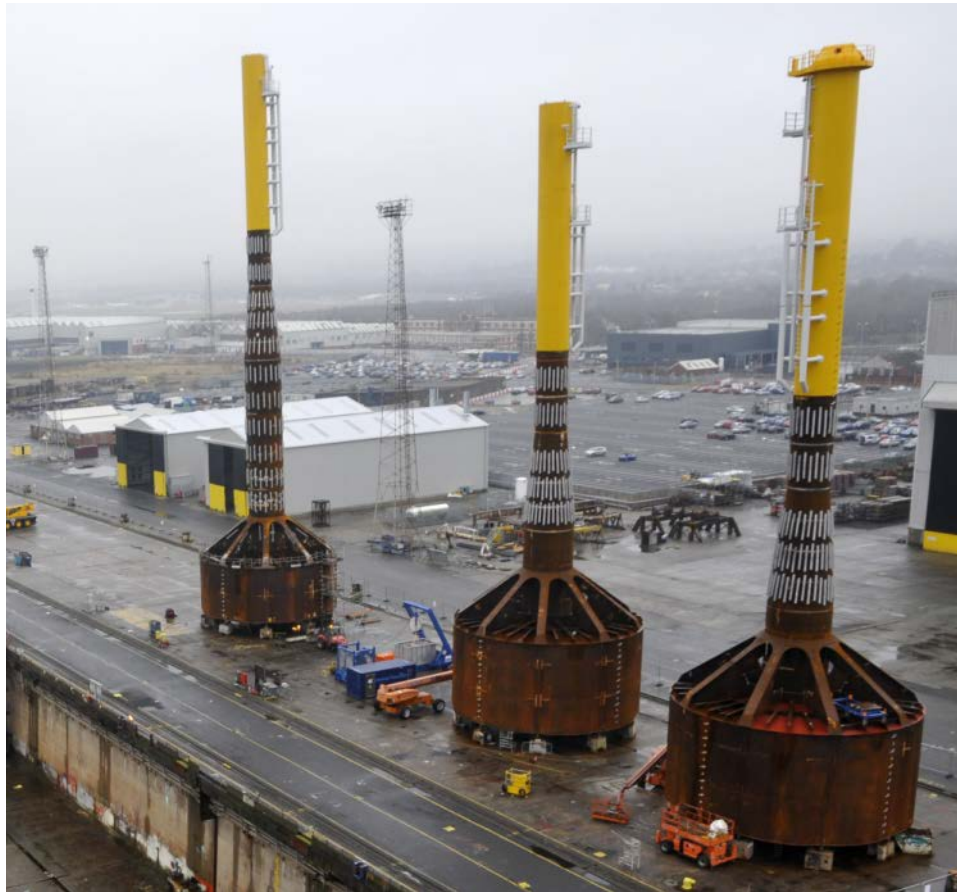
Figure 3-43: Suction Bucket Foundations for Dogger Bank and Firth of Forth Met Masts
