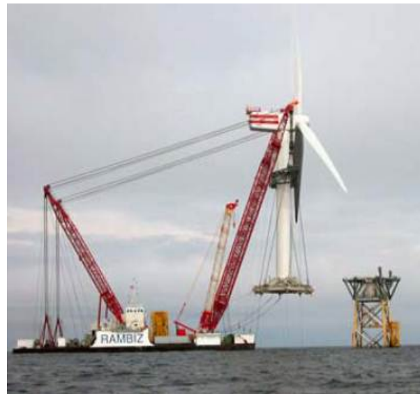
Figure 3-25: Installation of Fully Assembled REpower 5M Turbine at Beatrice
