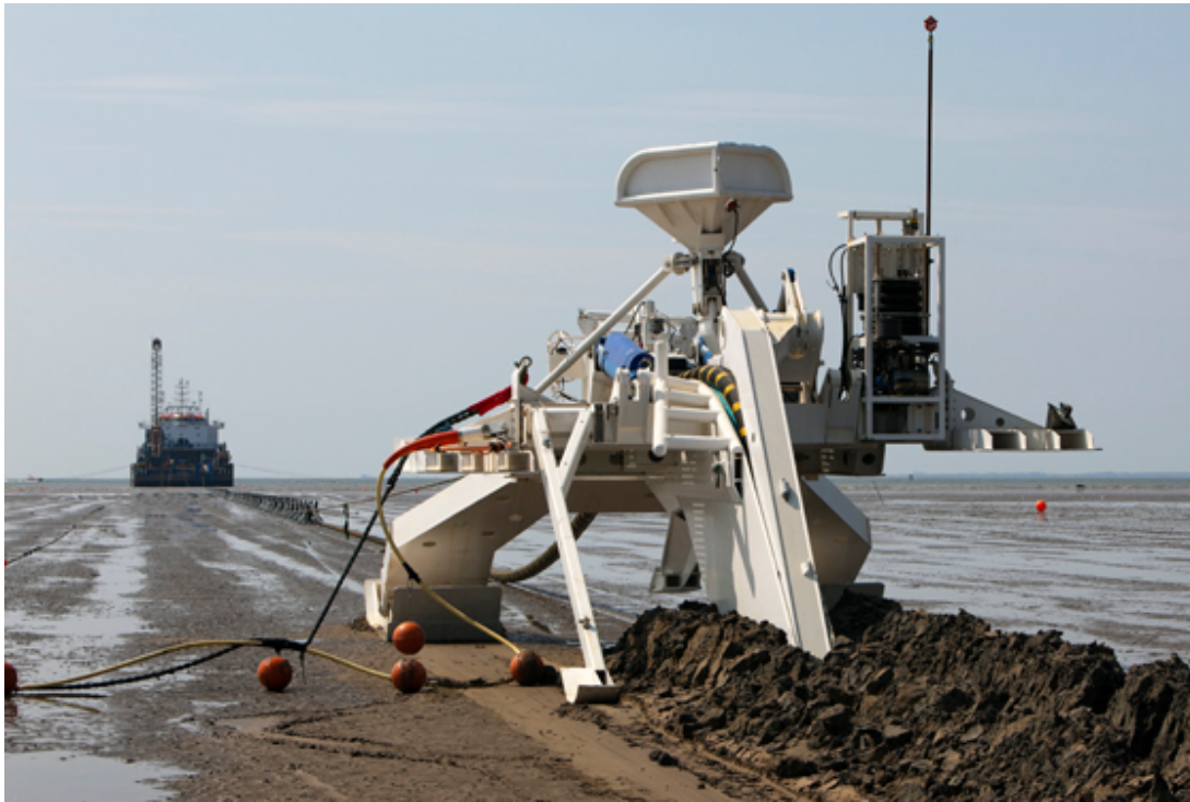
Figure 3-30: Visser & Smit Marine Contracting Sea Stallion 4 Subsea Cable Plow Burying Cable at the Shore
