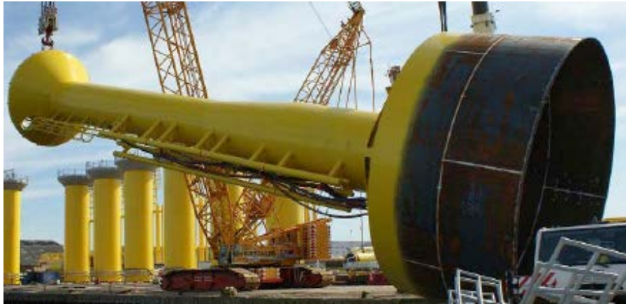
Figure 3-44: Suction Bucket Foundation
