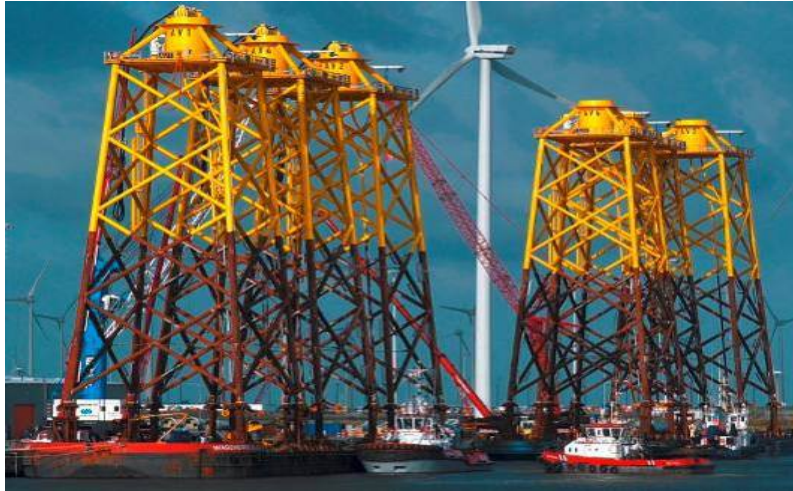
Figure 3-20: Jacket Structures on Barges Awaiting Installation in Pre-Piled Foundations
