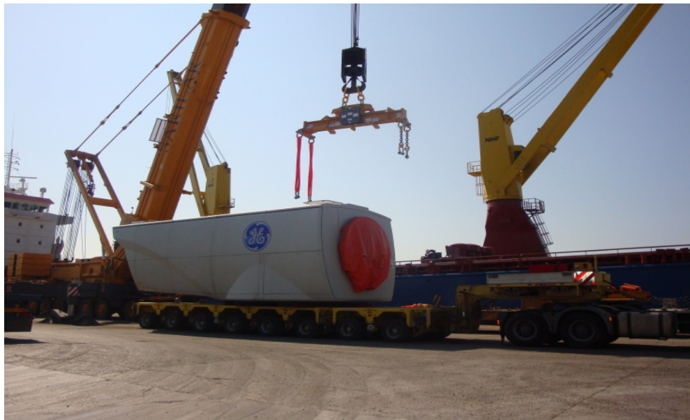
Figure 3-6: Spreader Bar for a Nacelle Lift Operation
