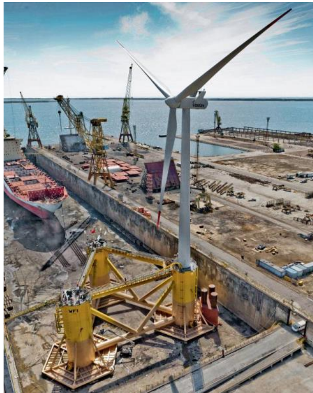
Figure 3-35: Principle Power's WindFloat Foundation and Vestas V80 Turbine Pre-assembled in a Dry Dock
