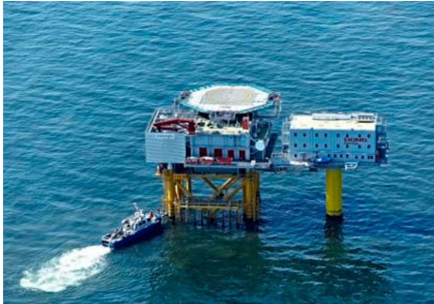
Figure 4-23: Accommodation Platform (right) and Substation (left) at Horns Rev 2 [28]
