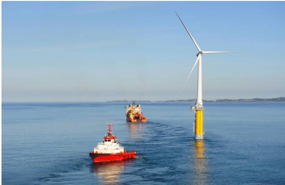
Figure 3-33: Float-out of Hywind Spar-class Foundation and Siemens 2.3 MW Turbine
