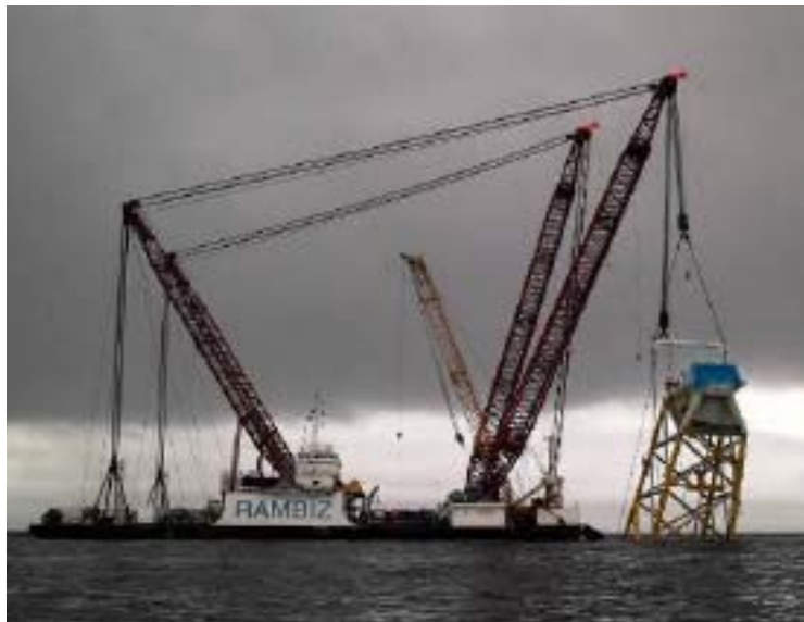
Figure 3-21: Rambiz Up-ending a Leg-Sleeved Jacket at Beatrice
