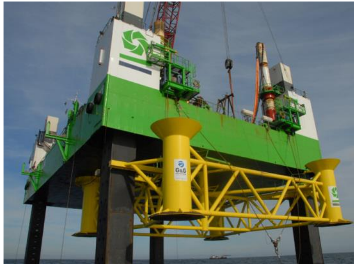
Figure 3-19: Piling Frame Used at Ormonde Slung Underneath GeoSea's Buzzard Jack-up Vessel
