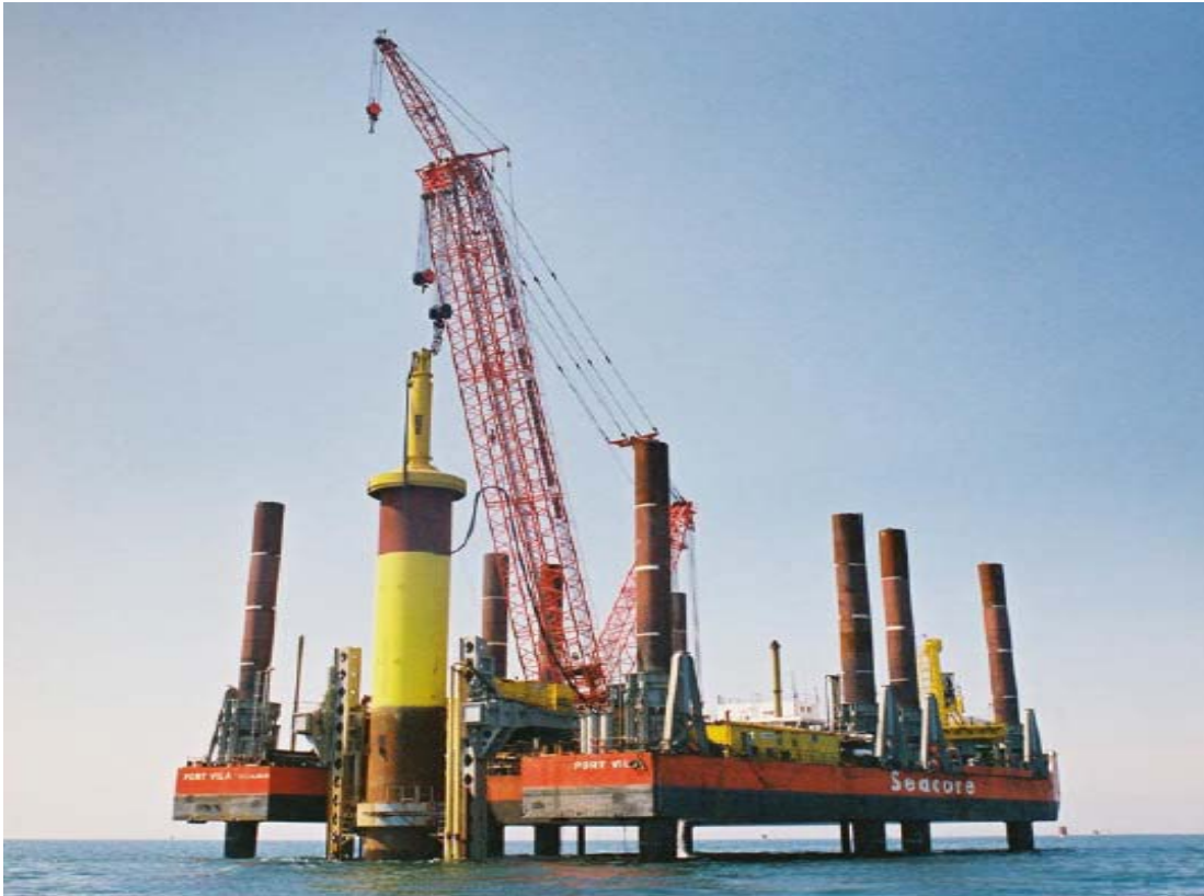
Figure 3-11: Steel Monopile being Driven by a Menck Hydrohammer – Jack-up Excalibur
