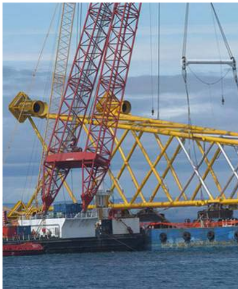
Figure 3-21: Rambiz Up-ending a Leg-Sleeved Jacket at Beatrice
