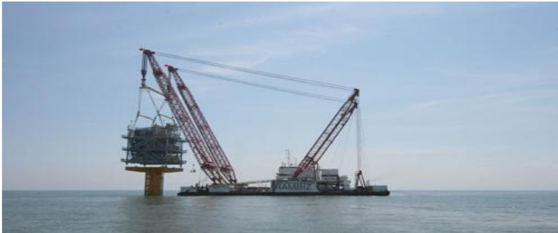
Figure 3-31: Substation Topside Installation at the London Array Project, UK
