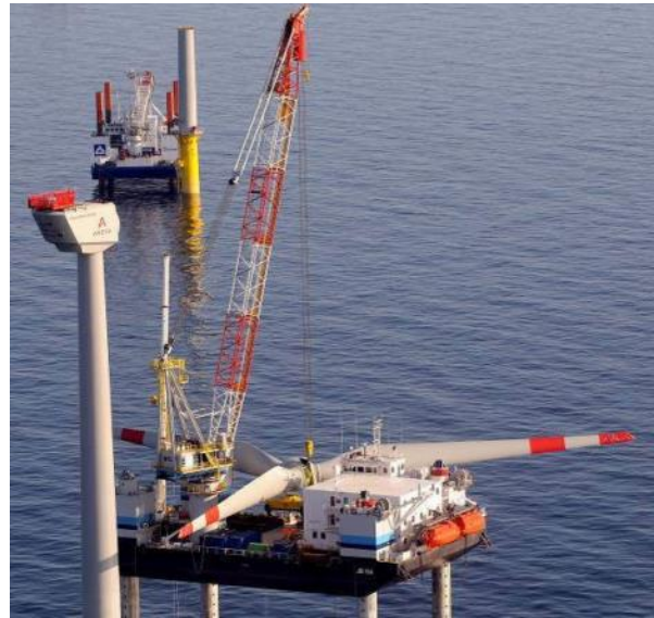
Figure 3-24: Full Rotor Assembly being Fitted to Areva Multibrid M5000 Nacelle
