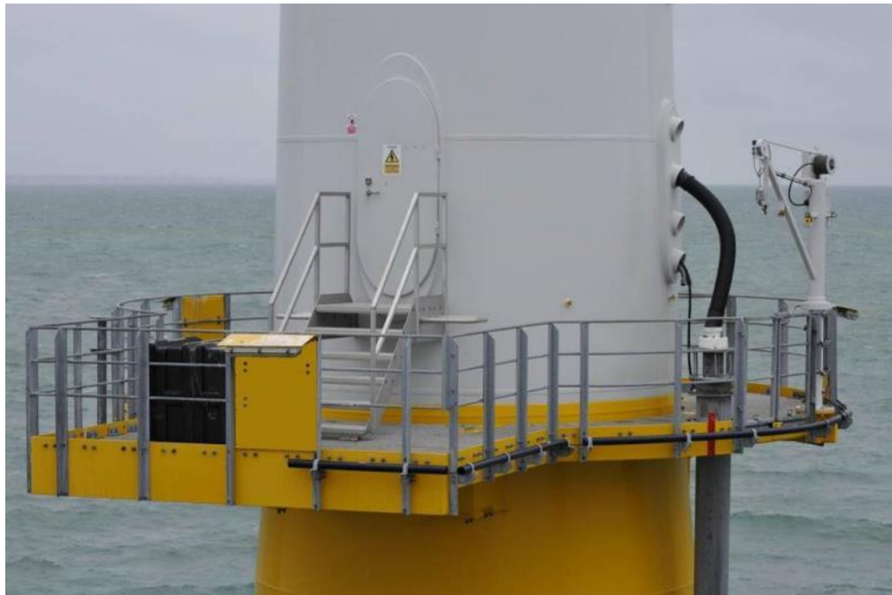
Figure 4-3: Platform and Davit at Top of Foundation / Base of Tower
