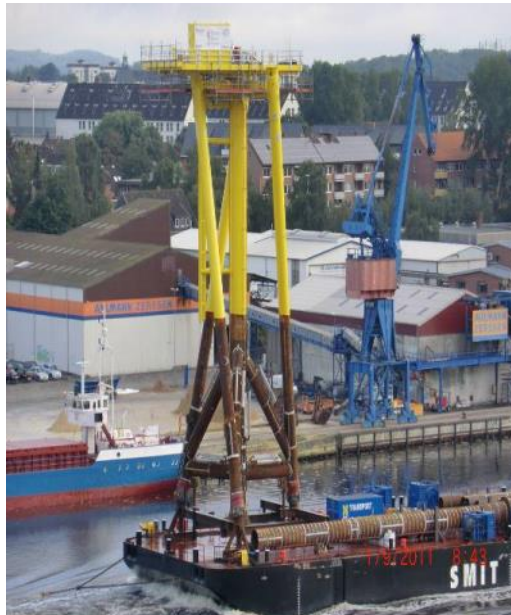
Figure 3-45: Keystone Engineering Inc Patented Inward-battered Guide Structure Technology and Hornsea Met Mast
