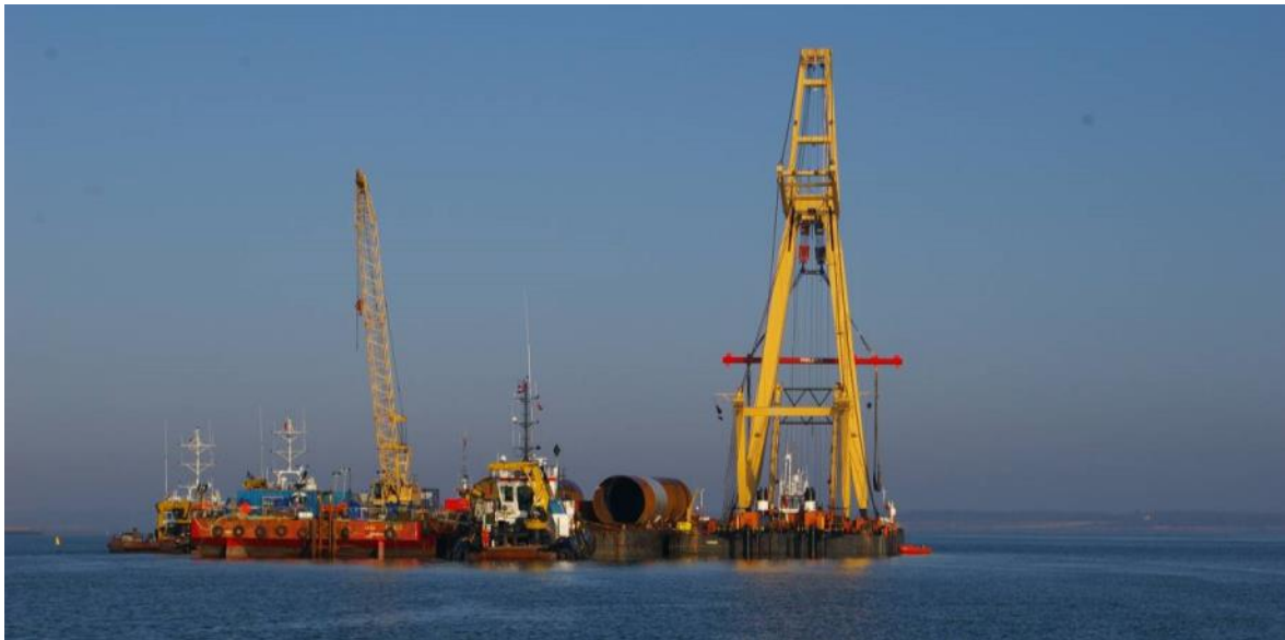
Figure 3-10: Monopiles Being Loaded onto a Deck Barge by Sheerleg Crane
