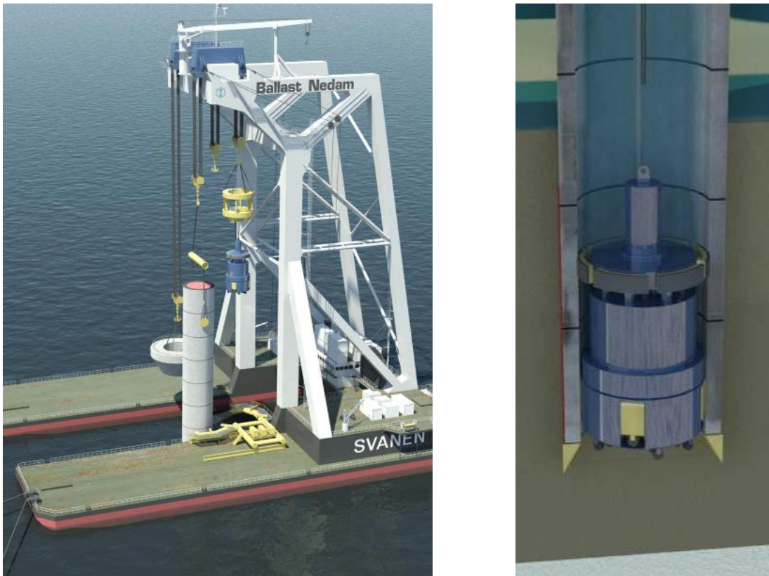
Figure 3-37: Installing Concrete Drilled Monopile – Svanen (vessel) and Detail of Drilling Plant
