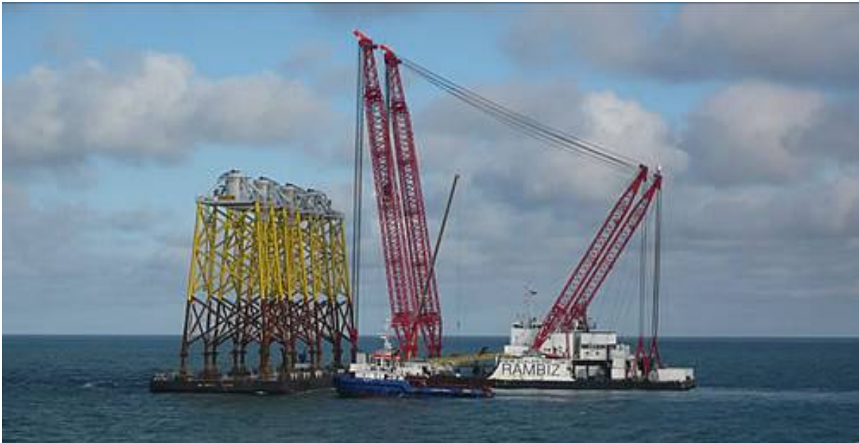
Figure 3-18: Scaldis Rambiz Offloading Jackets from a Deck Barge at Ormonde, UK
