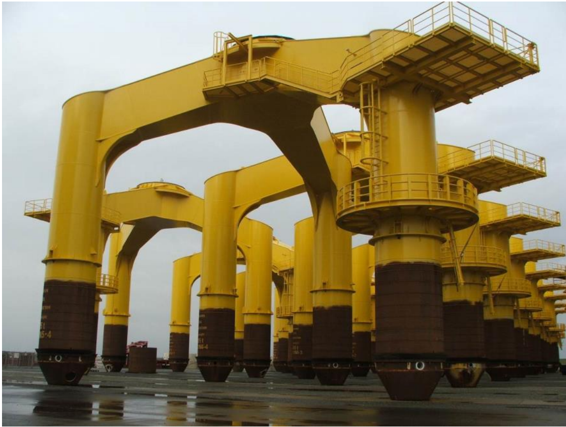
Figure 3-39: Tri-pile Foundations at Cuxhaven Steel Construction Awaiting Installation at BARD Offshore 1 in German North Sea
