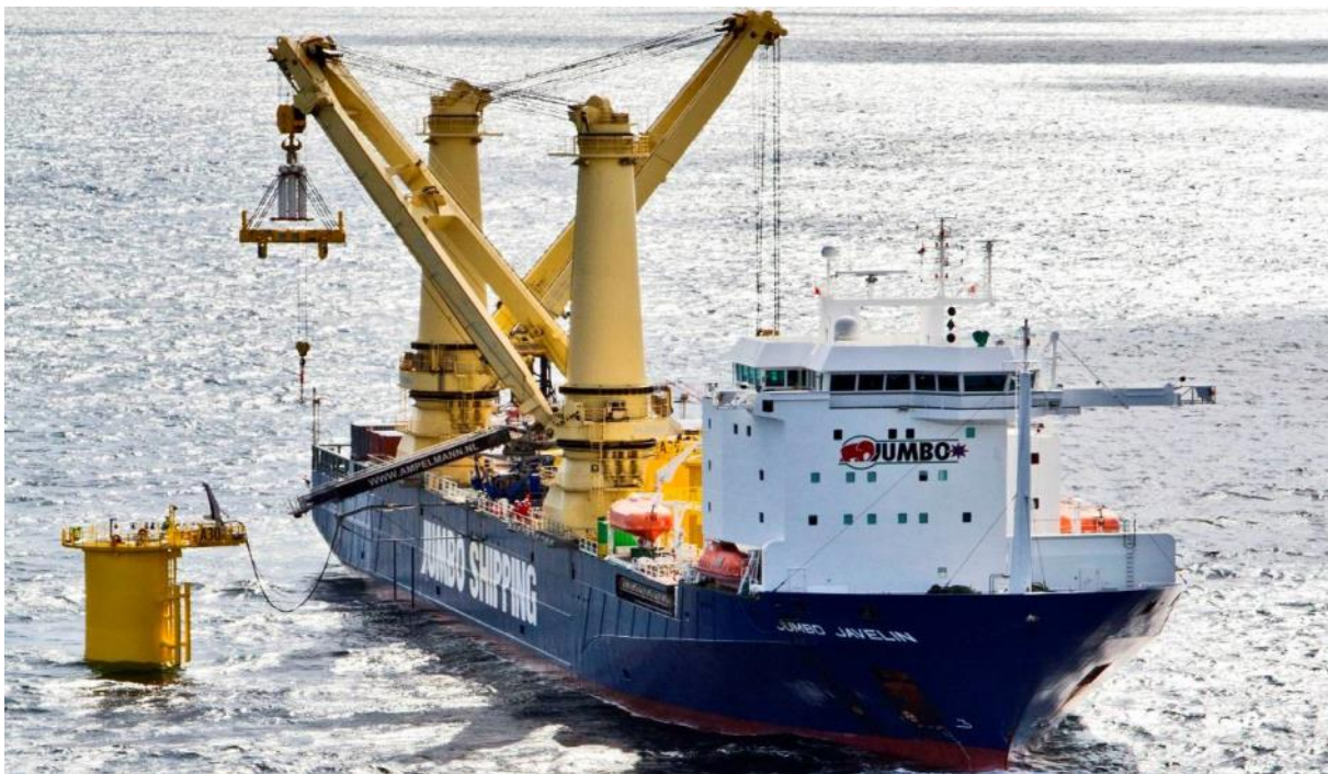
Figure 3-14: Jumbo Shipping Jumbo Javelin Heavy-lift Cargo Vessel Installing Transition Pieces and Grouting at the Anholt Offshore Project
