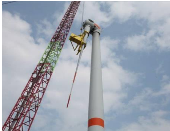
Figure 3-8: Turbine Blade Spreader Beam (yoke)
