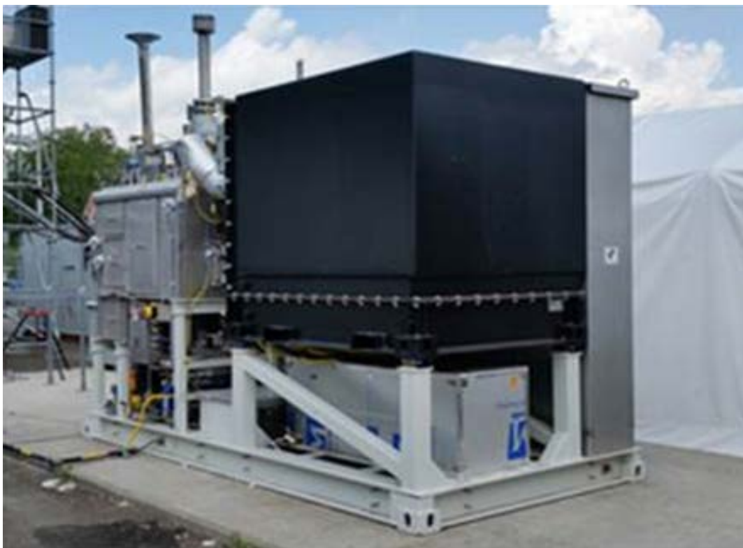
Figure 3-7. Module with Enclosure after Integration with BoP
