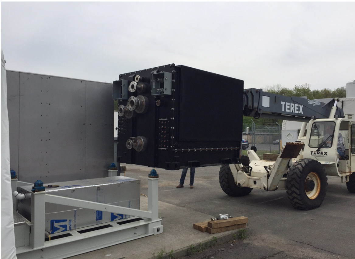
Figure 3-8. Installing Stack Module in 50 kW PCM Plant
