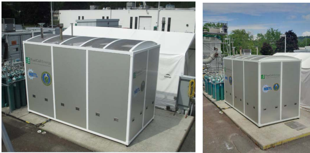
Figure 5-25 Façade Constructed around 50 kW PCM Plant
