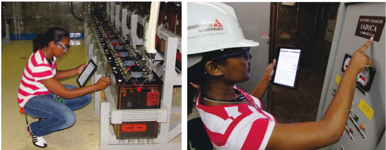
Figure 3. A maintenance technician at Plant Vogtle performs the battery and charger test and inspection work order.
