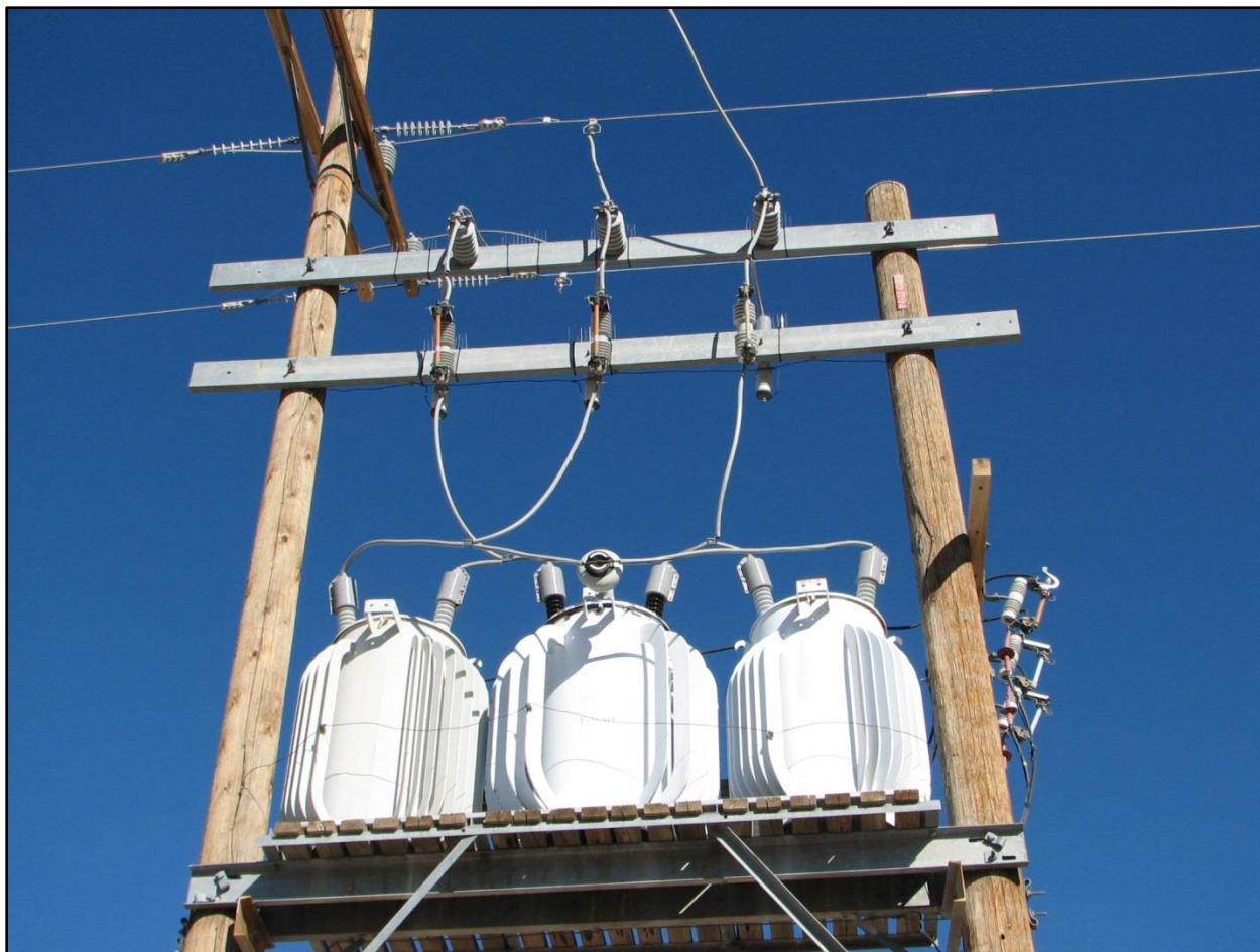
Figure 6-4. Retrofit pole with bird guard, insulator caps and metal spikes on crossarms at the Area 5 RWMC
