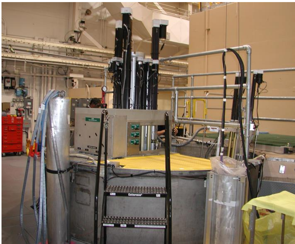
Figure 2. The ACRR Tank and High Bay.
