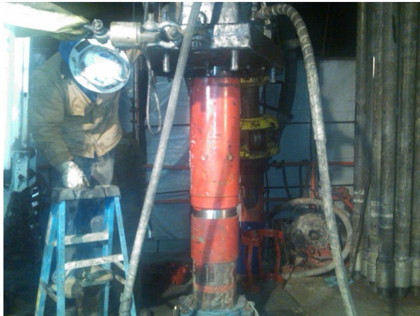
Figure 4.27. Installation of the 10 3/4-in. Multiple-Stage Cementing Collar
