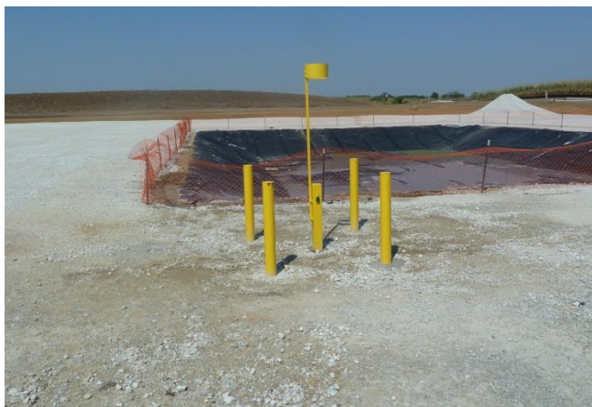
Figure 4.23. Shallow-Well Surface Completion
