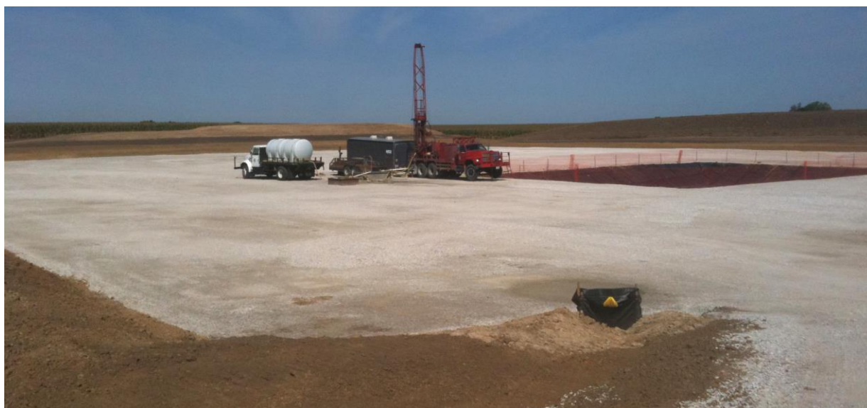
Figure 4.20. The FutureGen 2.0 CO 2 Storage Site Shallow Borehole Being Drilled Using a Mud-Rotary Rig. Fenced-off area to the right is the reserve mud pit for stratigraphic well FGA-1.
