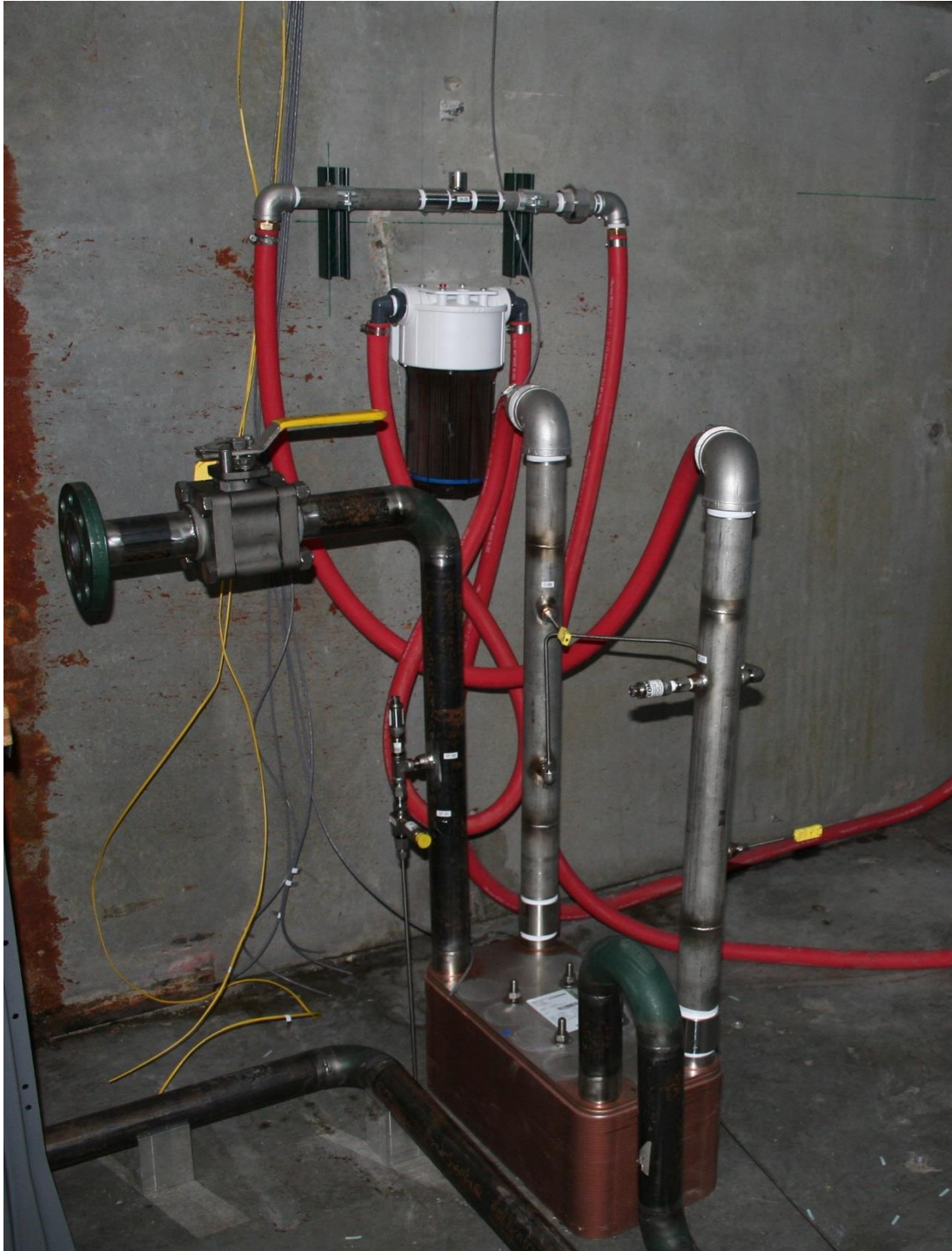
Figure 6. Heat exchanger (bottom of photo) along with piping and instruments. A water filter is mounted on the wall near the top.
