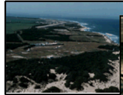
Kauai Test Facility Hawaii
