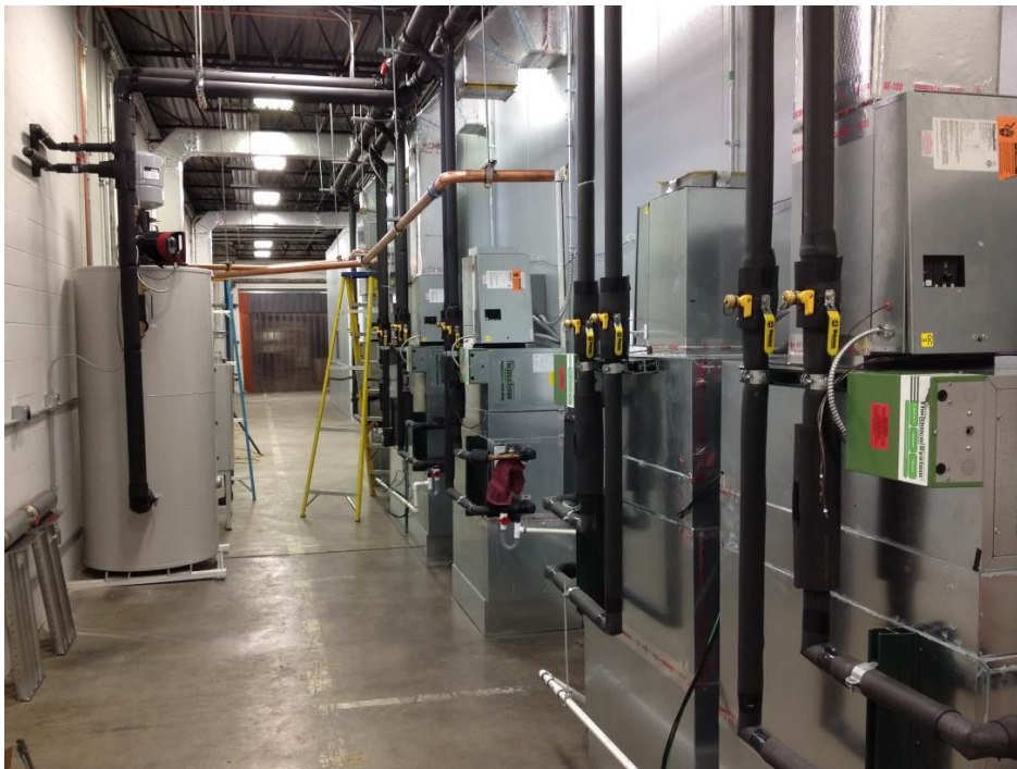
Figure 3: Backside of Chambers #2 and #3 showing the process equipment. The process control air handlers for the outdoor test cell are on the right. The chilled water storage tank is on the left.
