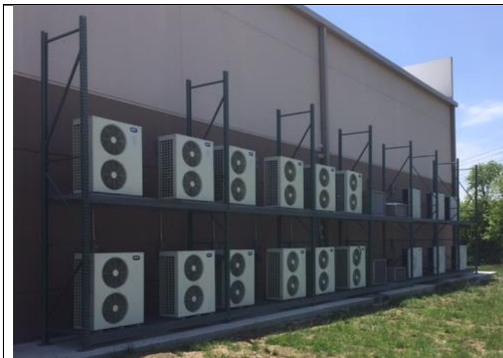
Figure 26 Outside of Lab. Racks and equipment: outdoor heat pumps and condensing units to condition the chambers and lab work space.
