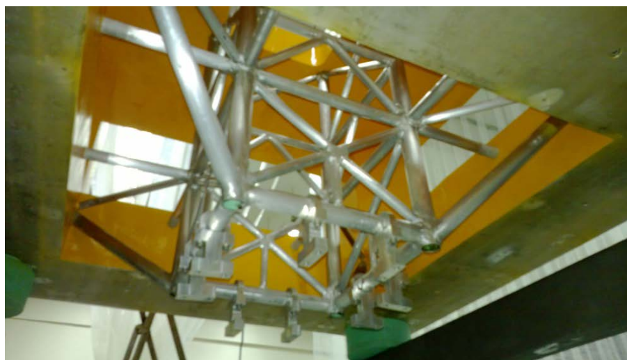
Figure 3-2. Hang-off structure installed in semi
