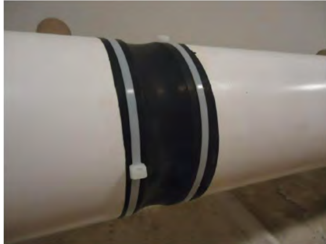
Figure 2-6 "Amazon" rubber sleeves sealing the interior between outer sheets.
