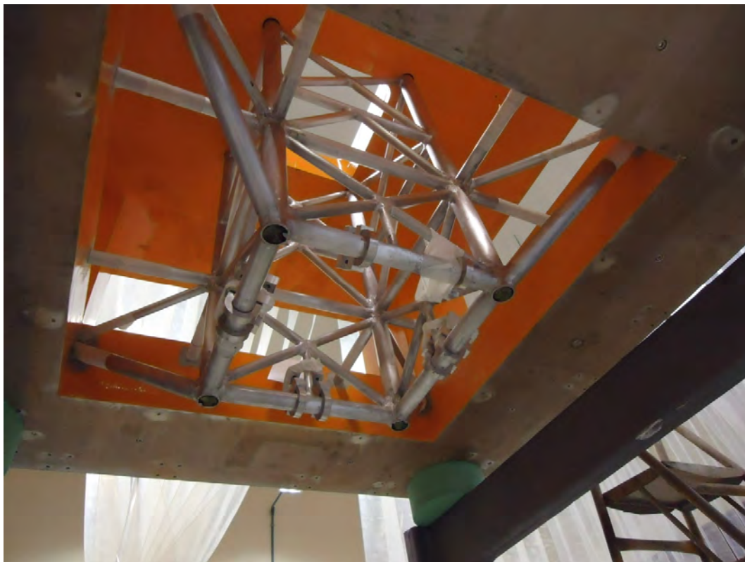
Figure 3-11 - CWP Hang-Off Frame Installed
