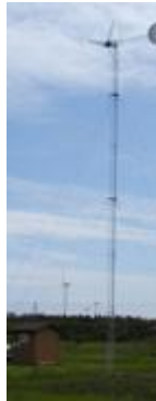
FIGURE 14: GUYED LATTICE TOWER
