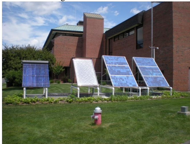
Figure 18, from left to right; Evacuated Tube Solar Collector, Flat Panel Solar Collector, and then the two Photovoltaic Arrays
