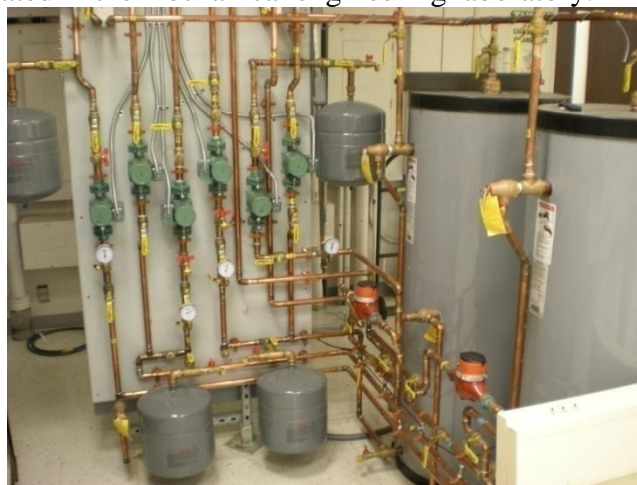
Figure 20, solar pipe network, heat exchangers, and mixing tanks in ME lab
