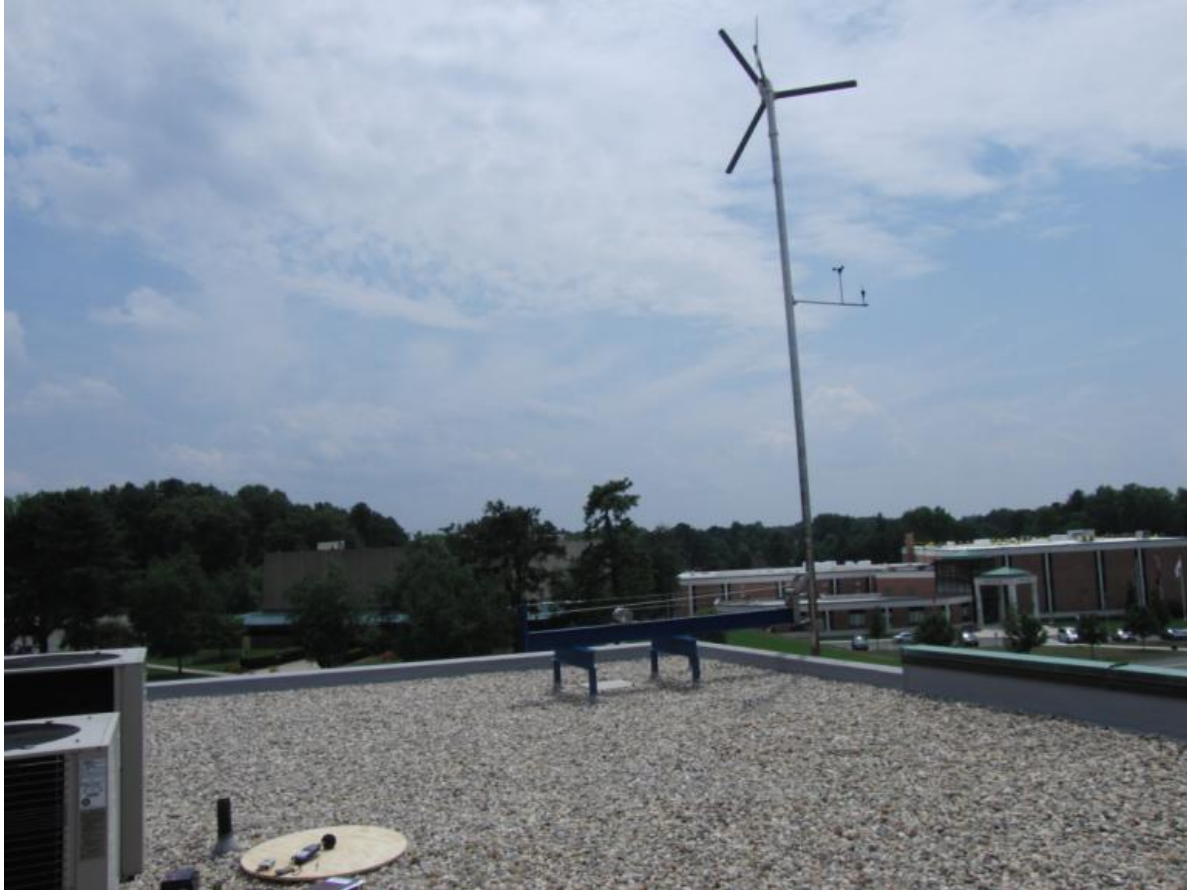
FIGURE 21: VIEW FROM THE ROOF OF SLEITH HALL OF THE BERGEY 1 KW WIND TURBINE ATTACHED TO THE SIDE OF SLEITH HALL AT WESTERN NEW ENGLAND COLLEGE.
