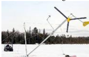
FIGURE 15: TILT-UP TOWER
