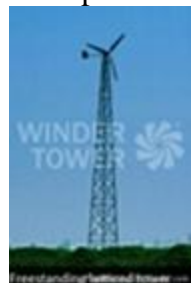
FIGURE 13: FREESTANDING LATTICE TOWER
