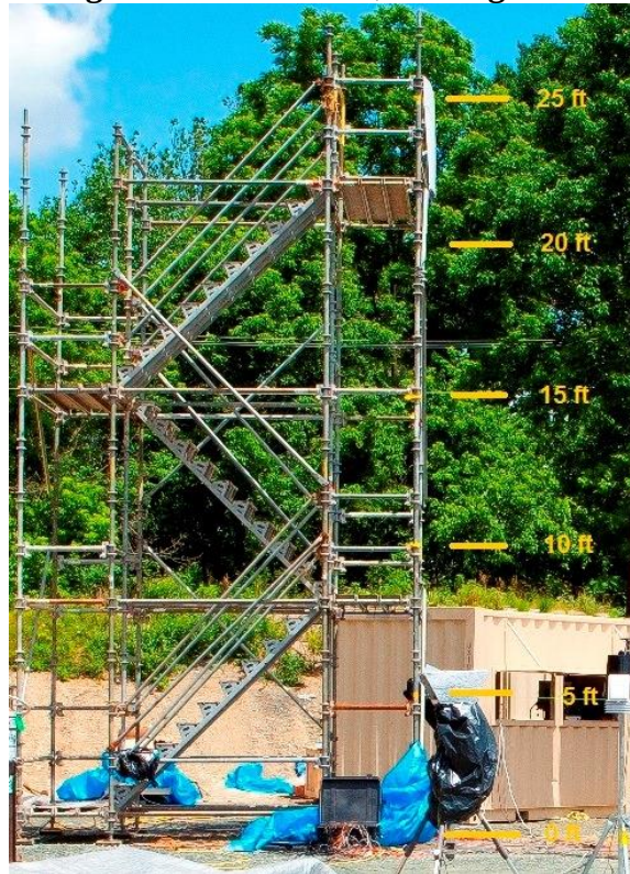
Figure 29. Close-up of the 26-ft (7.9-m) tall scaffold and creek bank trees.
