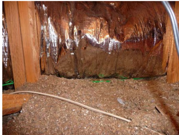
Figure 5. Duct section PA located about three feet downstream of supply plenum prior to insulation
