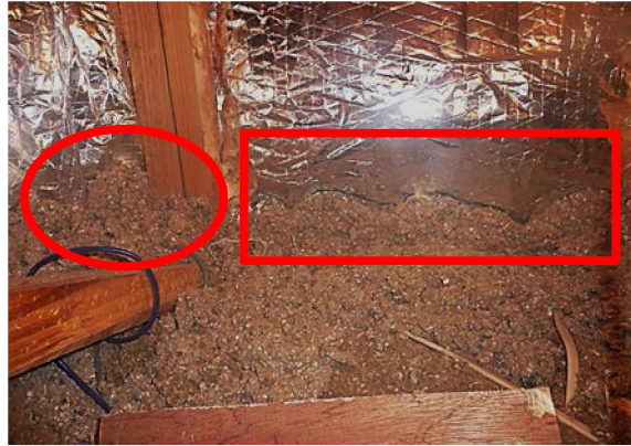
Figure 6. Duct section PA after insulation wrap has been installed. In the red rectangle, the foil facing will be tucked under and cellulose added. In the red circle, the foil facing has been tucked under, and a small amount of cellulose insulation has been added where the duct wrap meets the existing cellulose.
