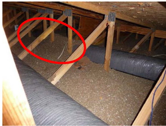
Figure 4. Flex duct section 8A partially covered by attic insulation prior to being wrapped with insulation
