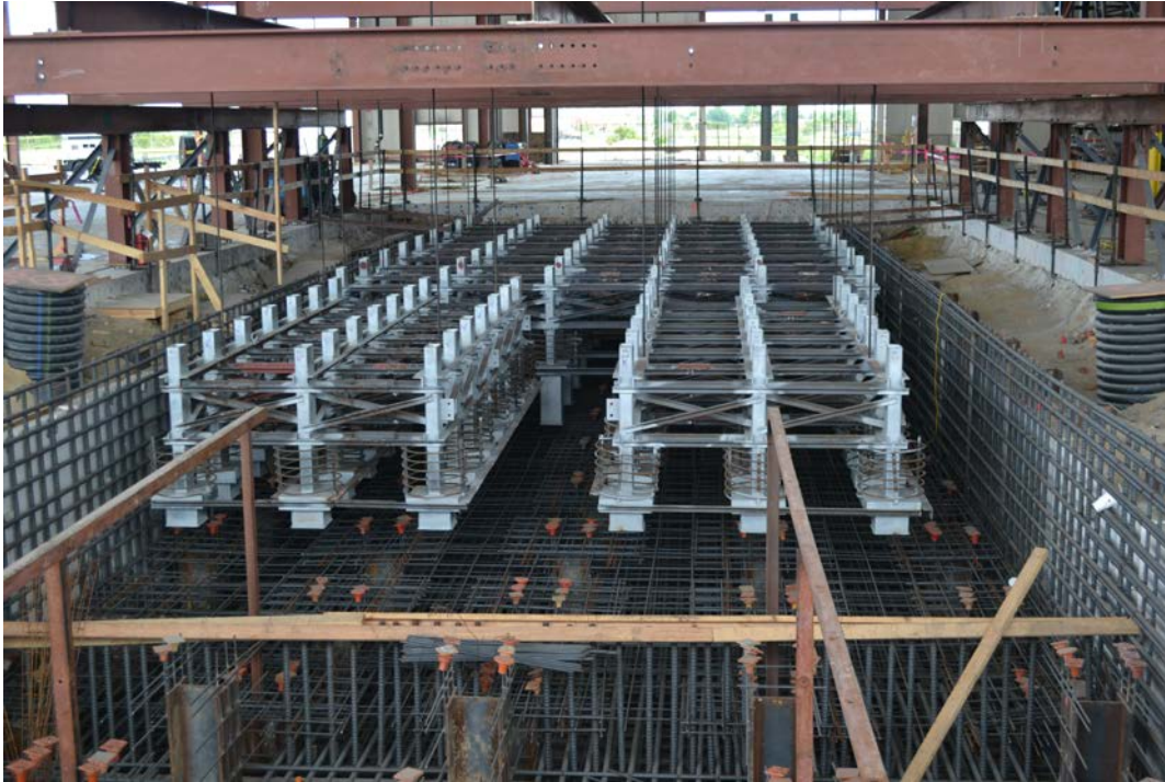
Figure 21 7.5 MW Foundation Anchor Embedment's
