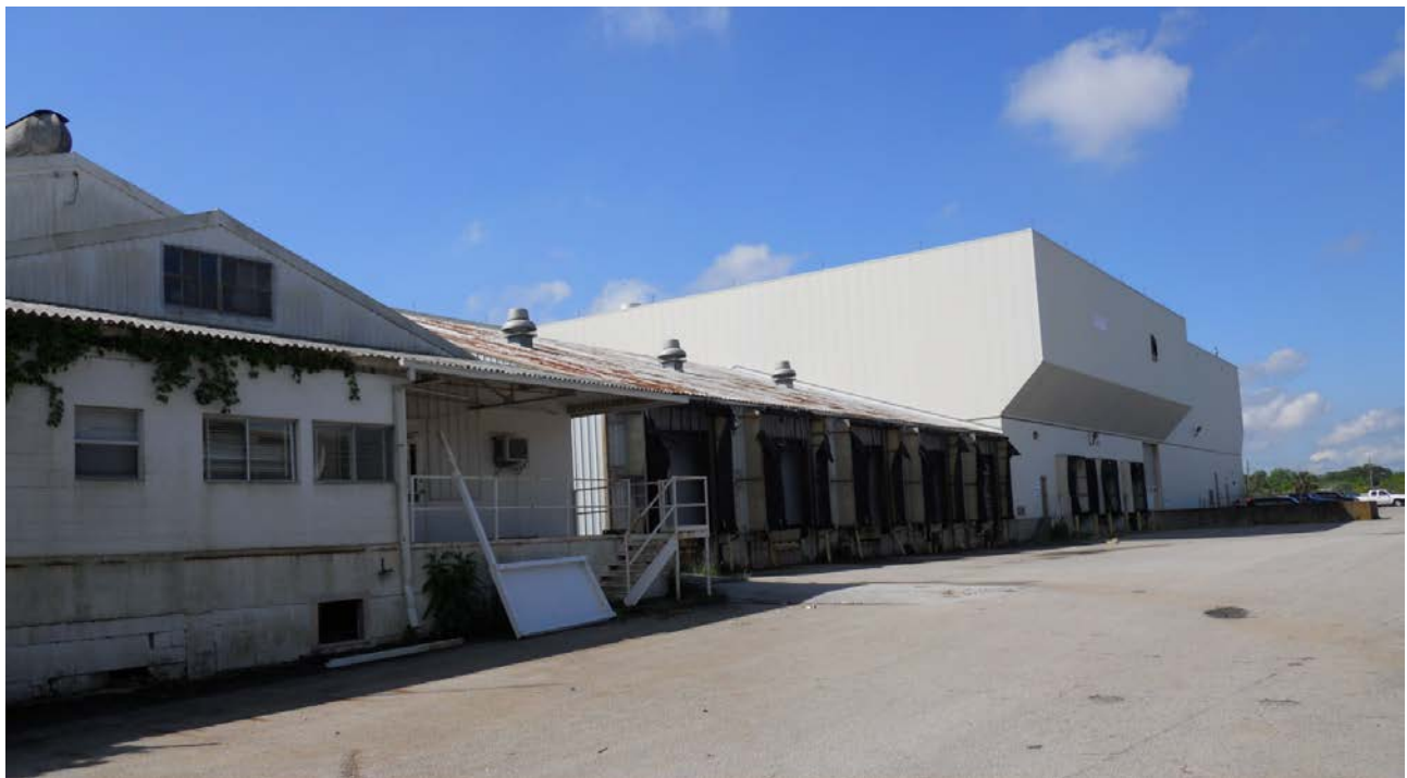
Figure 2 Building 69 Exterior Prior To Renovation
