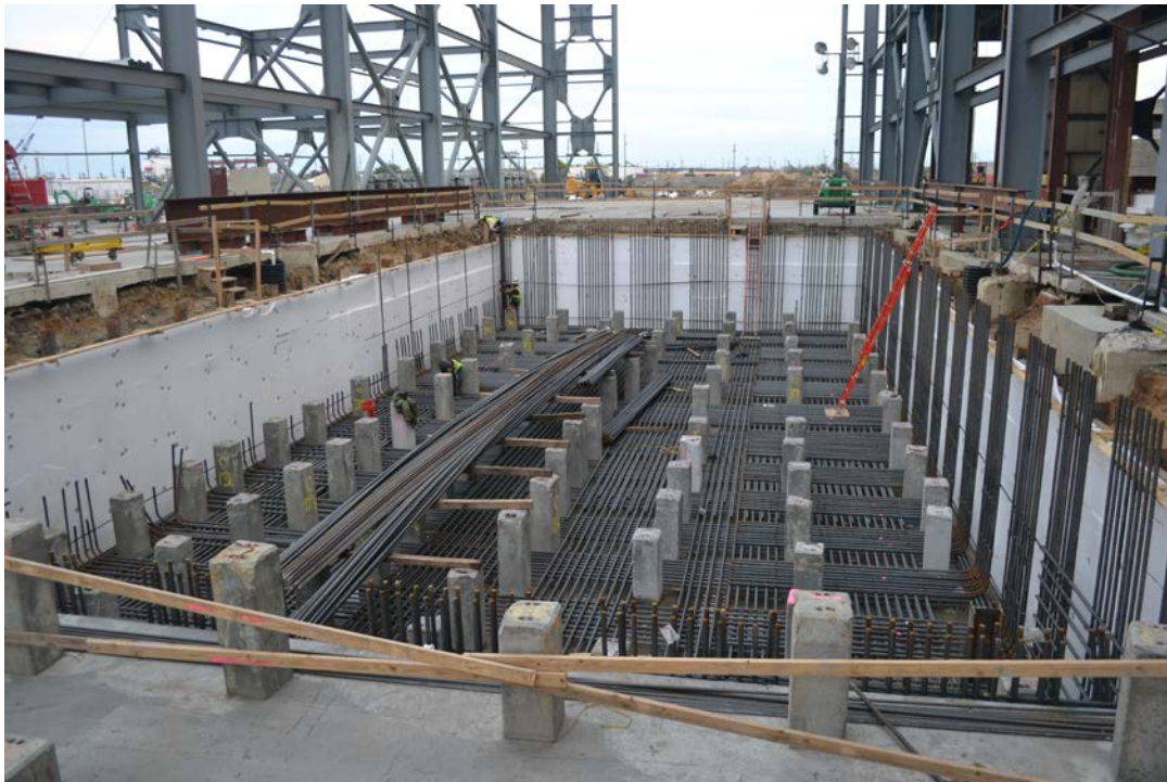
Figure 22 Pilings and Base Layer of 15 MW Foundation with Isolating Wall
