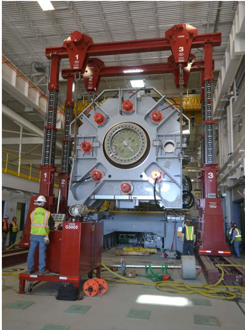
Figure 33 Portable Gantry Crane Lift of 7.5MW LAU
