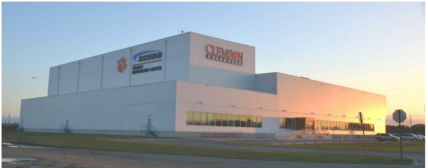
Figure 9 Front Façade of Renovated EIC Facility
