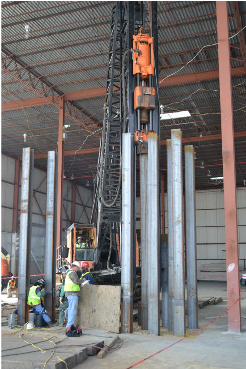
Figure 19 New Piles for Structural Pilecap
