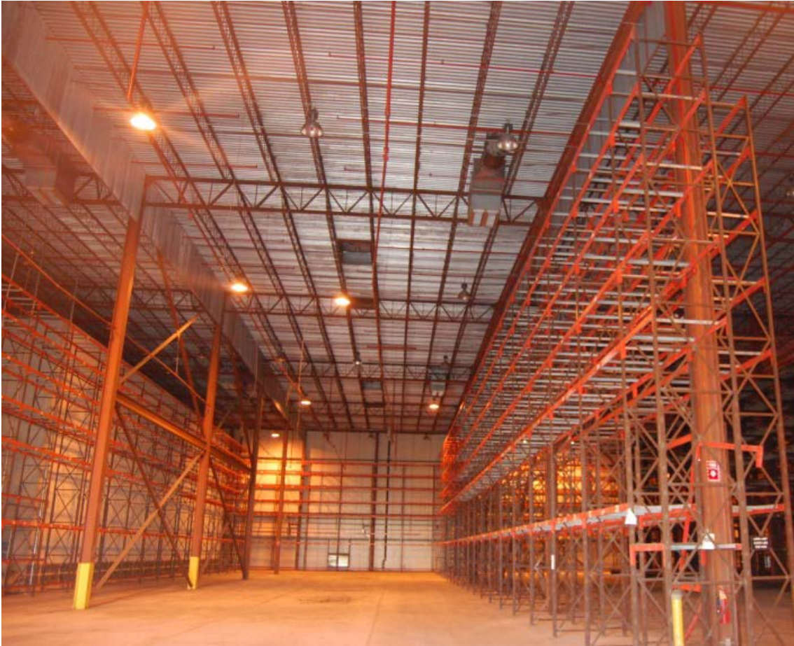
Figure 3 Building 69 Interior Prior To Renovation
