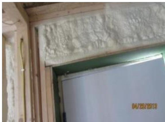
Figure 12. Reductions in framing around the openings allows for more insulation in headers.
