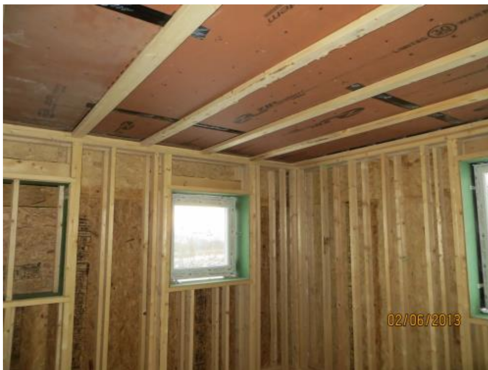
Figure 1. Double-wall construction
