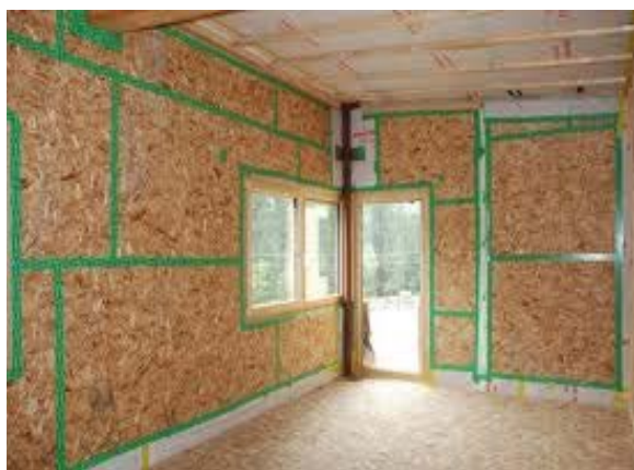
Figure 14. Interior air barrier with all seams taped
