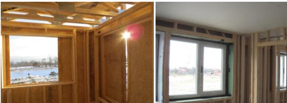
Figure 13. Windows in double walls: (left) a framed window opening and (right) a set window
