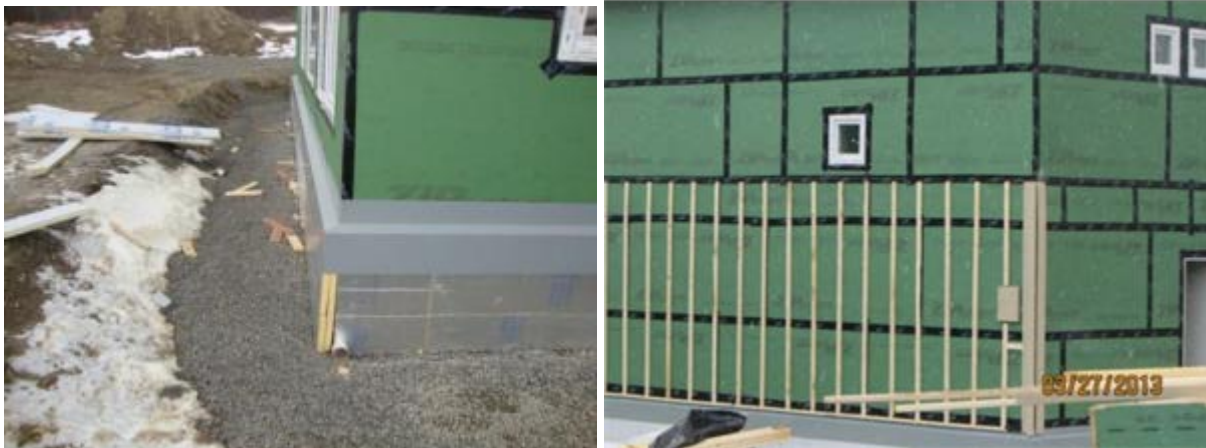
Figure 8. Flashing over slab edge insulation was taped to the sheathing using the manufacturer's approved tape. The vented cladding was then attached with \frac{3}{4} -in. furring strips, and it overlapped the flashing.
