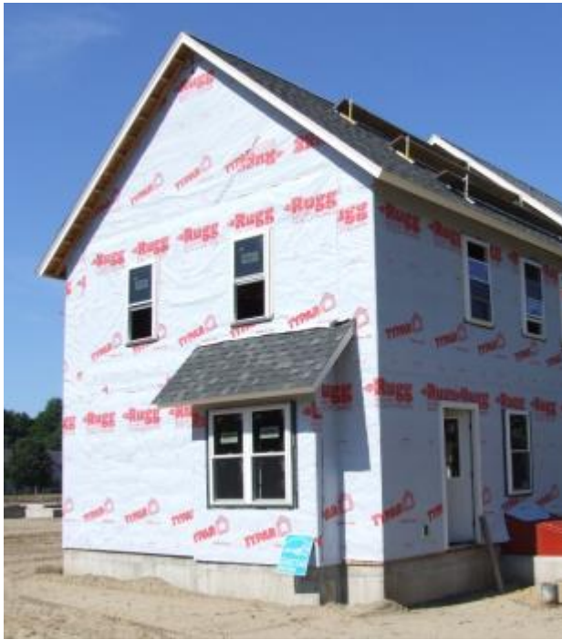
Figure 18. Example of a building wrap being used for the WRB
