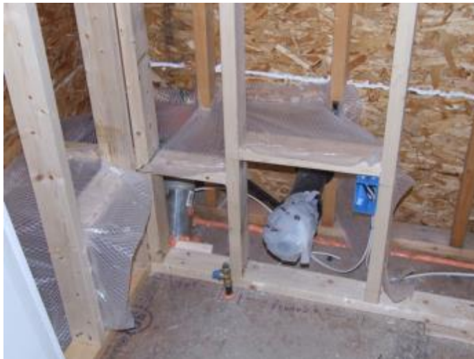
Figure 9. Insulation netting surrounds vents and plumbing penetrations in an exterior double wall.
