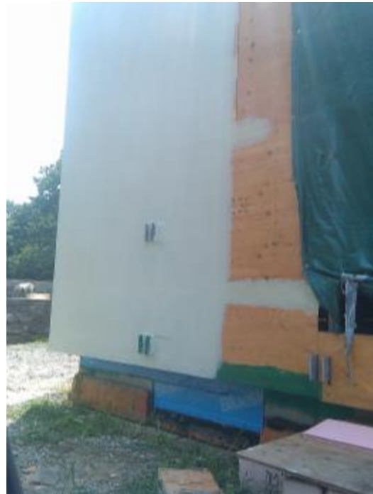
Figure 19. Image of liquid-applied WRB
