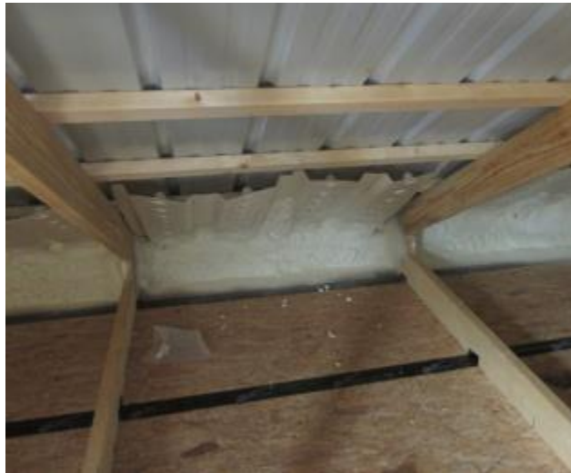
Figure 7. ccSPF installed over the outer edge of the double wall to the desired R-value for the ceiling
