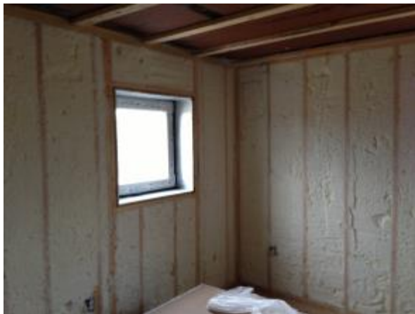
Figure 2. ocSPF in a 12-in. double wall
