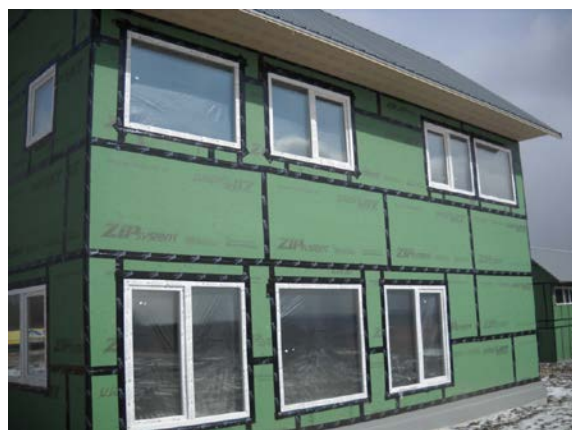
Figure 15. Exterior air barrier with all seams taped
