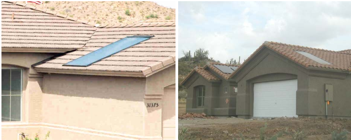
Figure 14. RITH 4 (left) and RITH 5 (right) installations.
