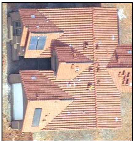
Figure 1: Aerial view of both systems installed on the Calnex model home in the Phoenix area. Notice the dormer causes some shading in the morning on the PV panels.
