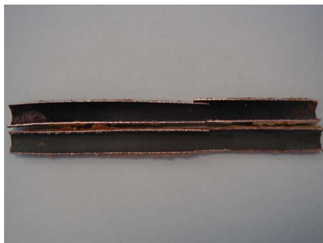
Figure 15. Copper tube leading to the tank inlet shown in Figures 13 and 14.
