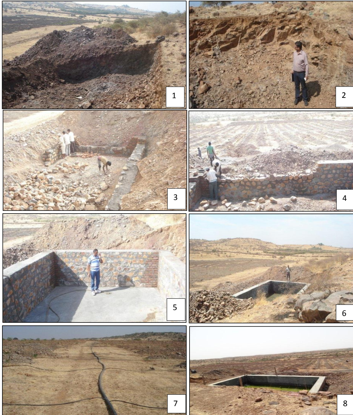
Figure 46. Making of reservoir for gravity irrigation system:
