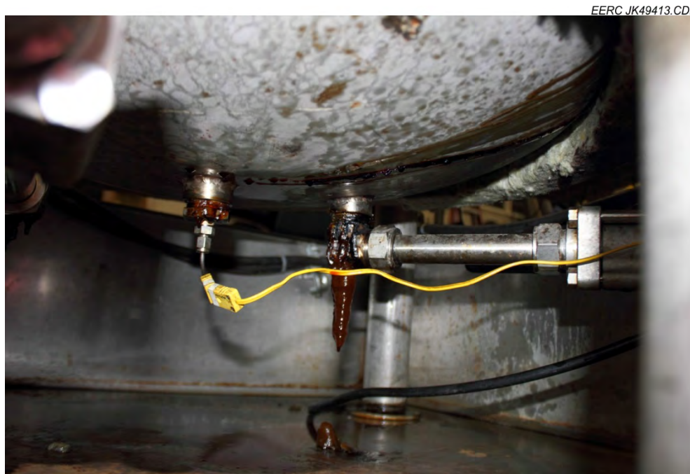
Figure 4-6. Solvent leaks at the base of the stripper column.
