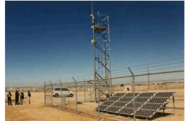
Outdoor Test Facility
