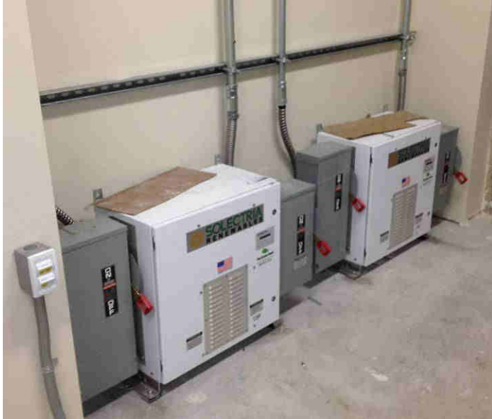
Solar PV inverters.
