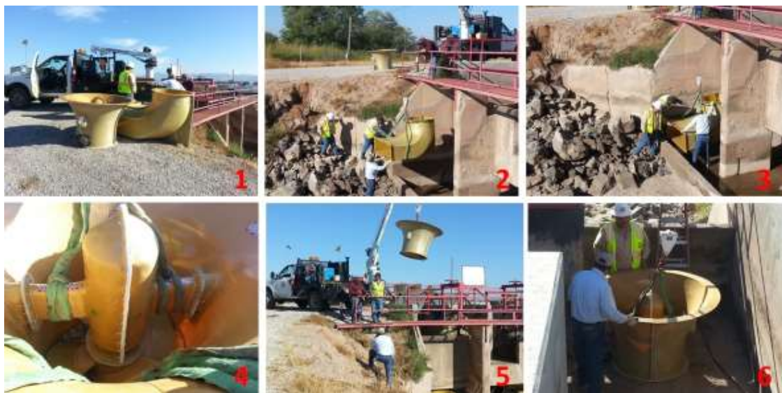
Figure 8. 1) Turbine modules ready for installation at the Drop 8 Station; 2) Hoisting the discharge module; 3) Placing the discharge module under the drop orifice; 4) Bracing the turbine; 5) Hoisting the turbine; 6) Placing the turbine above orifice
