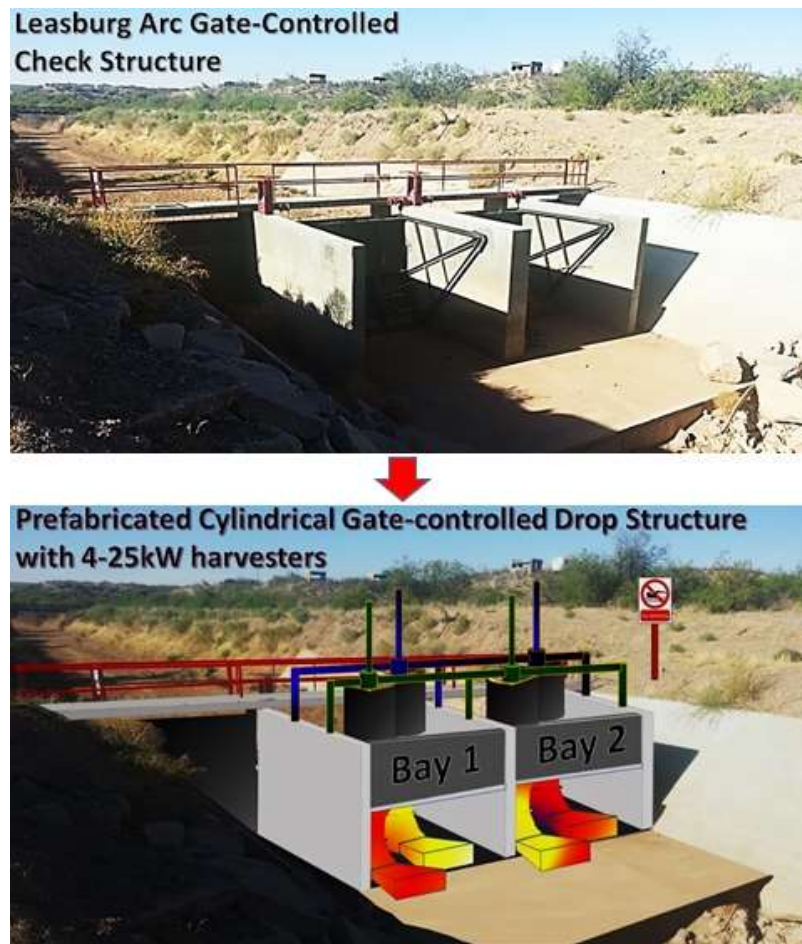
Figure 3. Possibility to transform a check structure into a drop structure
