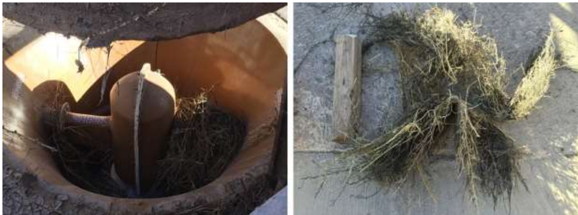
Figure 17. Debris clogging the turbine
