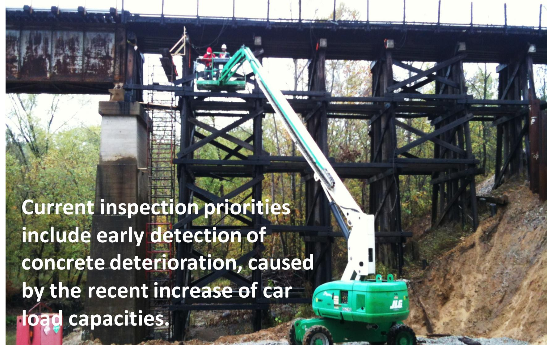
Current inspection priorities include early detection of concrete deterioration, caused by the recent increase of car load capacities.
