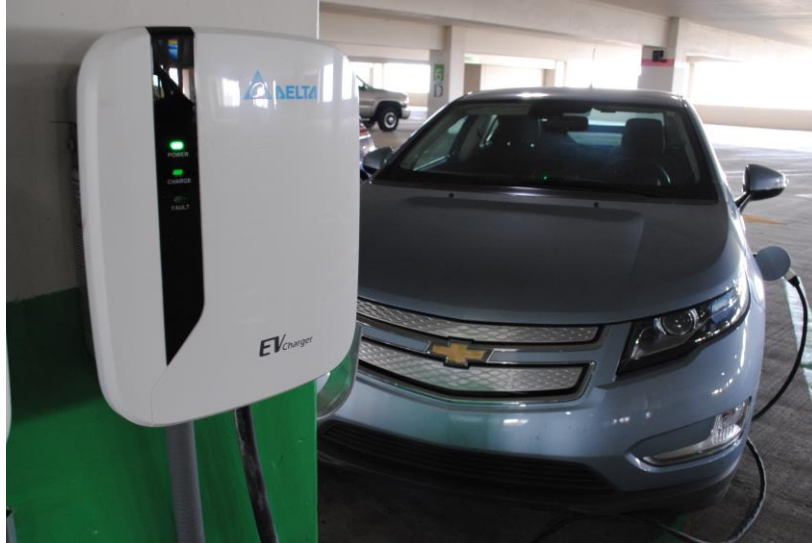
Figure 13: Photo of the 2 nd generation EVSE Prototype installed and under field trial at DTE's parking garage in downtown Detroit, MI. (Photo taken October 30, 2014)
