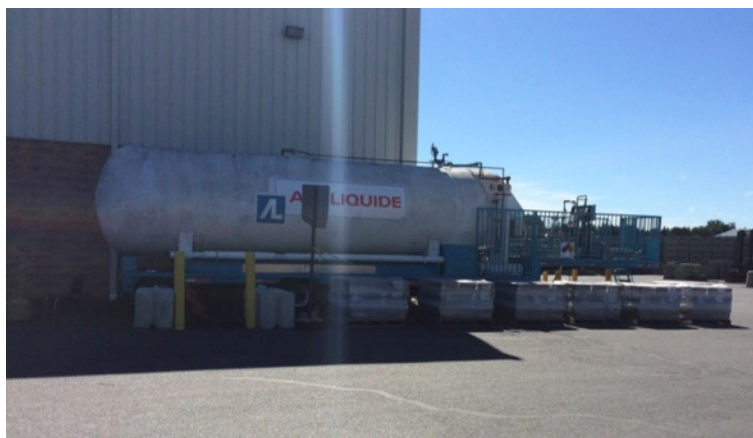
Figure 55. Temporary CO 2 tank
