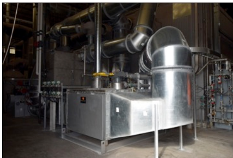
Figure 53. Gas conditioning system - view from heater
