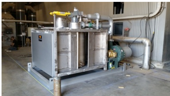
Figure 52. Gas conditioning system - heater
