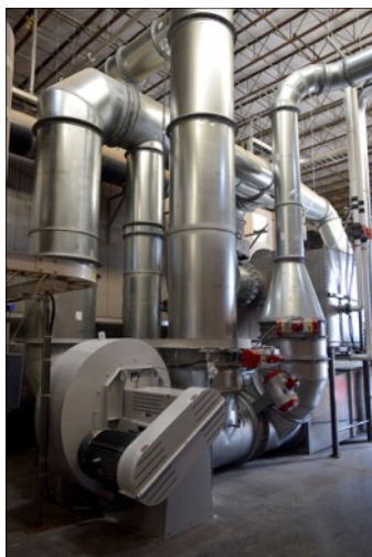
Figure 54. Gas conditioning system - view from side opposite heater
