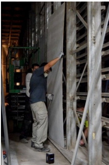
Figure 43. Magnesium oxide board installation
