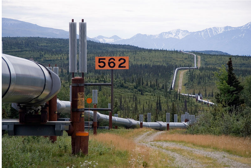
Figure D.1: Thermosyphons installed next to the trans-Alaska Pipeline [Wikipedia, 2011]
