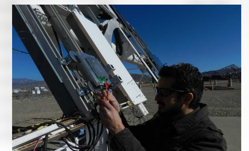
Attachment and connection of module to tracker
