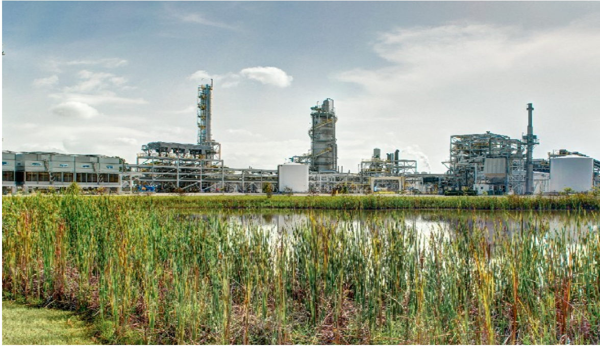
Figure 1 The facility utilizes a unique combination of gasification and fermentation processes using vegetative and yard waste from the local Indian River County to produce bioethanol and renewable power.
