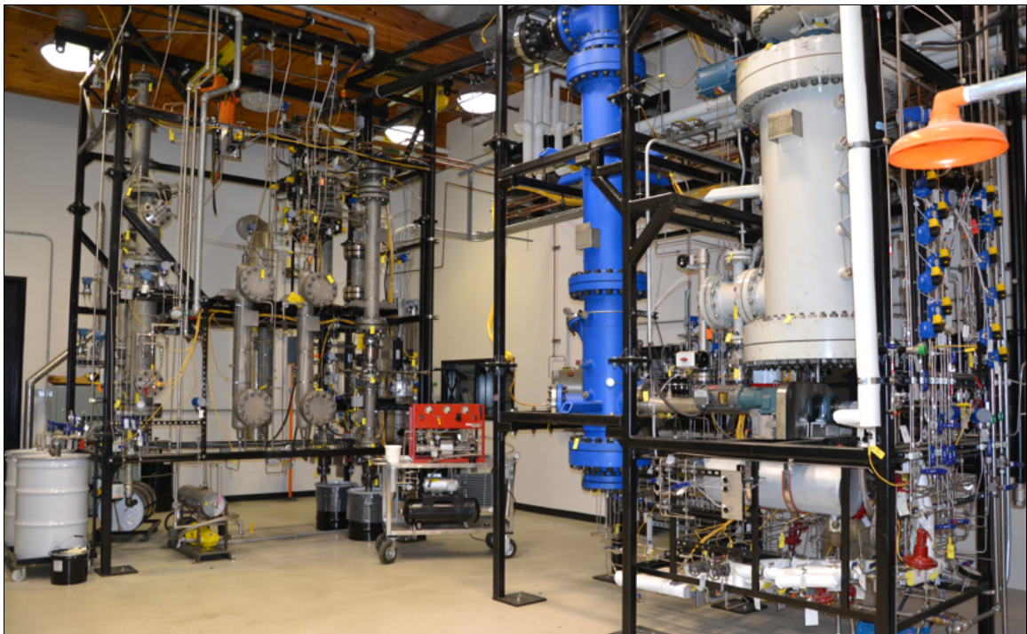
Auburn University's fluidized bed gasification and gas conditioning system.
