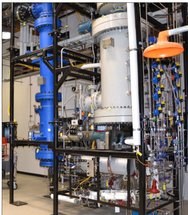
Gasification platform. Feed hoppers are shown on the right (white steel vessels) and gasifier is shown on the left (blue vessel).
