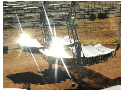
Dish Collectors at Sandia
