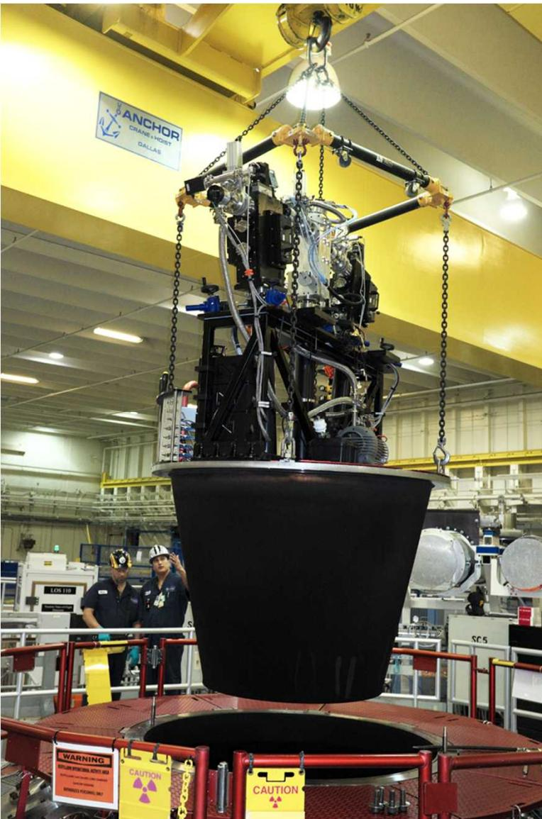
The array of opacity spectrometers is lowered into place with a 20 ton crane
