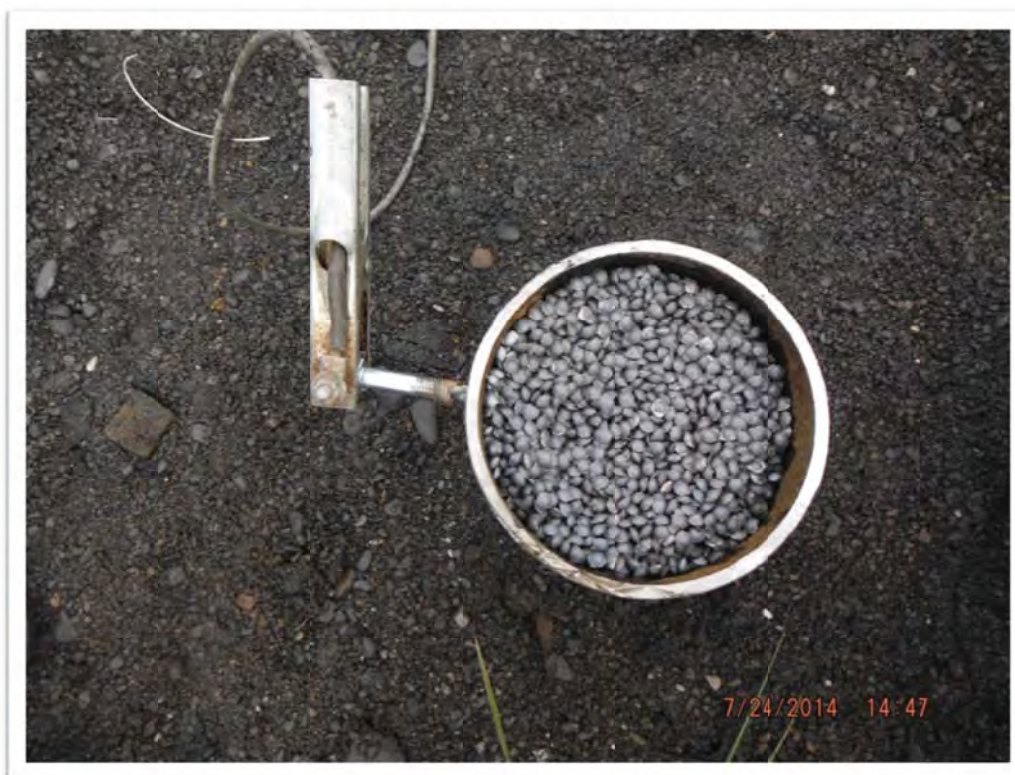
Photograph 10 – The casing interiors were sealed with a bentonite plug. A ground wire was attached to a bolt welded onto the left side of casing to allow welding of cap.
