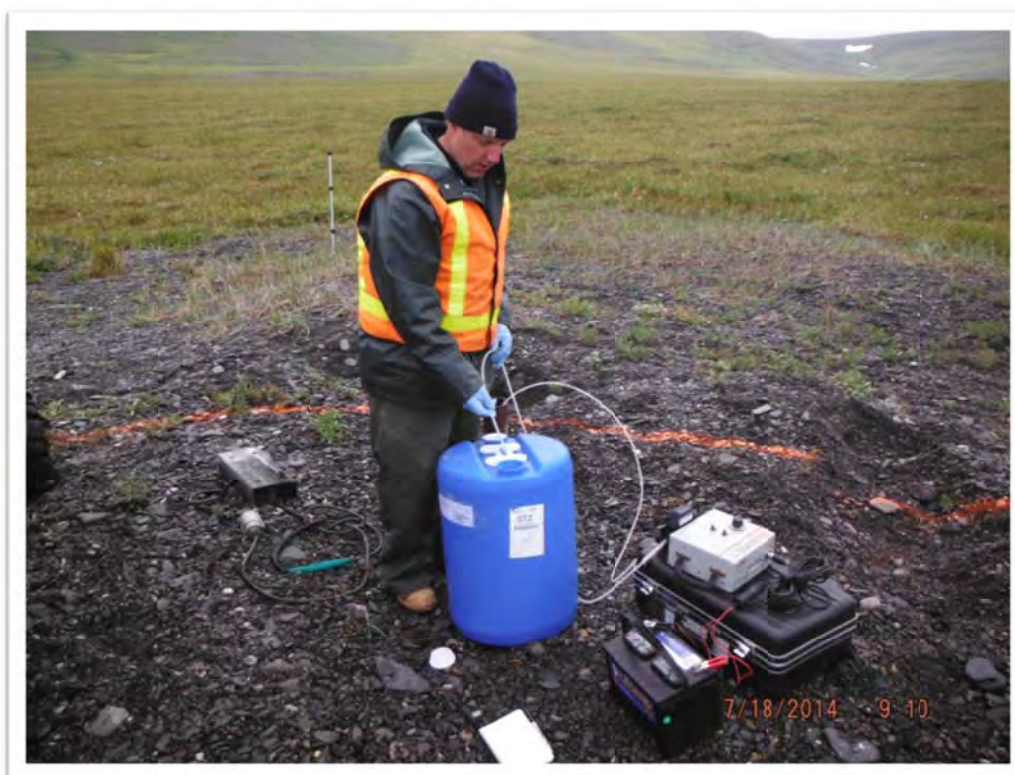
Photograph 22 – Standing water was pumped from the Test Hole Charlie casing prior to decommissioning and excavation activities. View to northwest.
