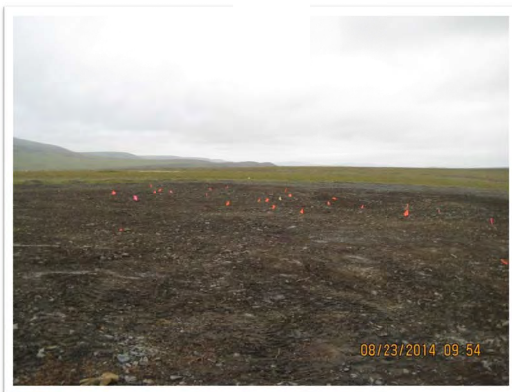
Photograph 52 – Test Hole X-1 following remedial action efforts. Pin flags marking confirmation samples locations were re-installed using swing-ties. View to southeast.
