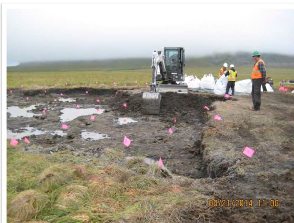
Photograph 38 – Limits of Test Hole Dog excavation with pin flags marking the floor and wall PID screening locations. View to the west.
