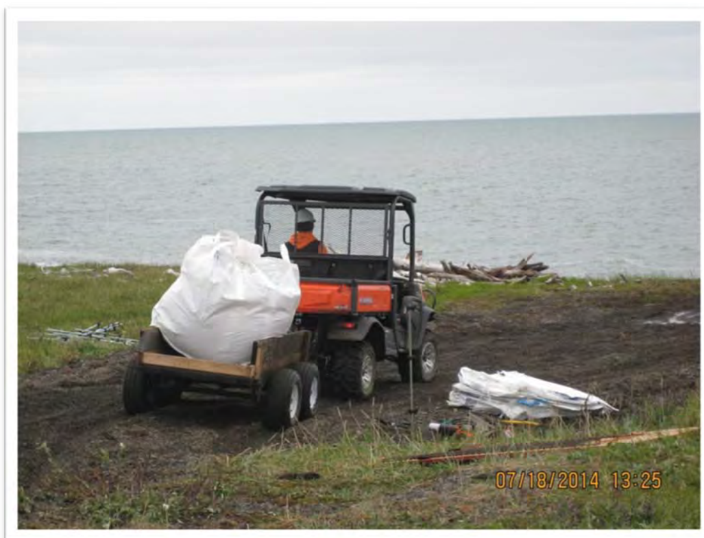
Photograph 53 – Filled super sacks were transported to staging area on trailers pulled by ATVs or UTVs (shown here). View to south.
