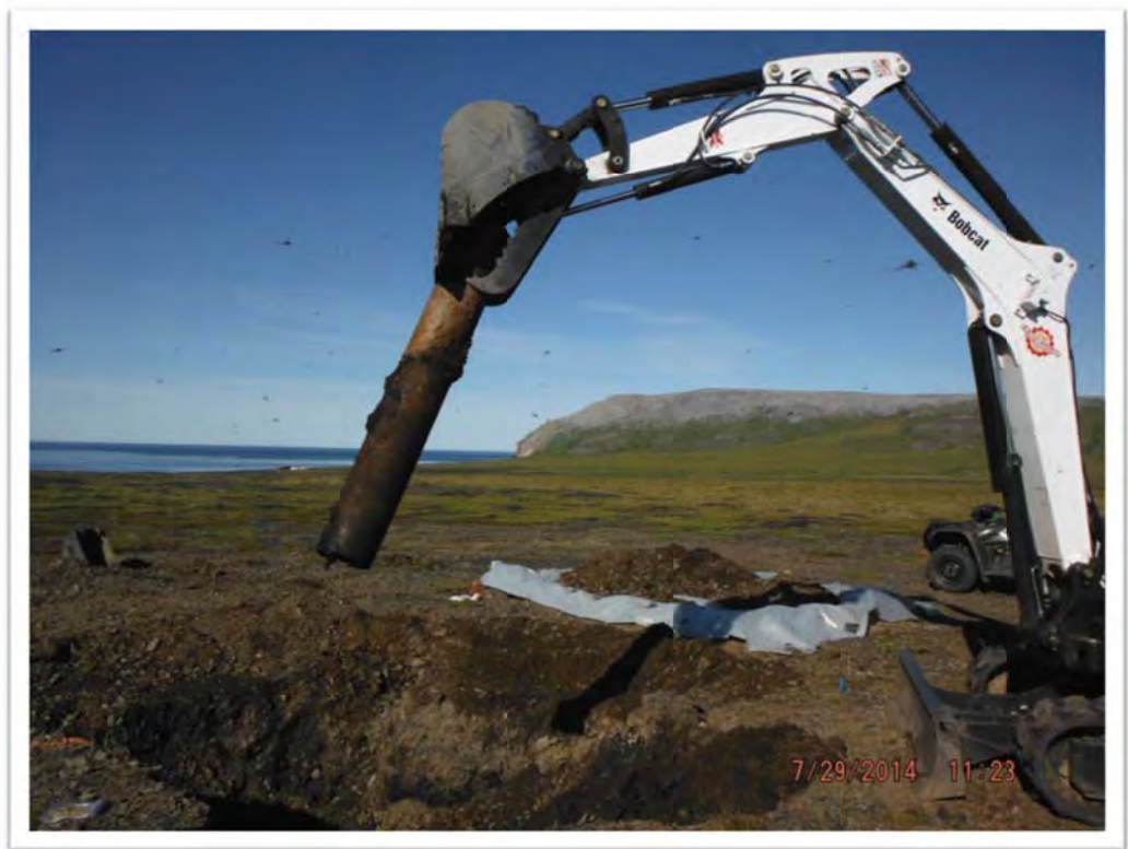
Photograph 44 – The 6-foot-long Test Hole X-1 casing was completely removed. Stockpiled surface soils are shown on far side of excavation. View to the west.
