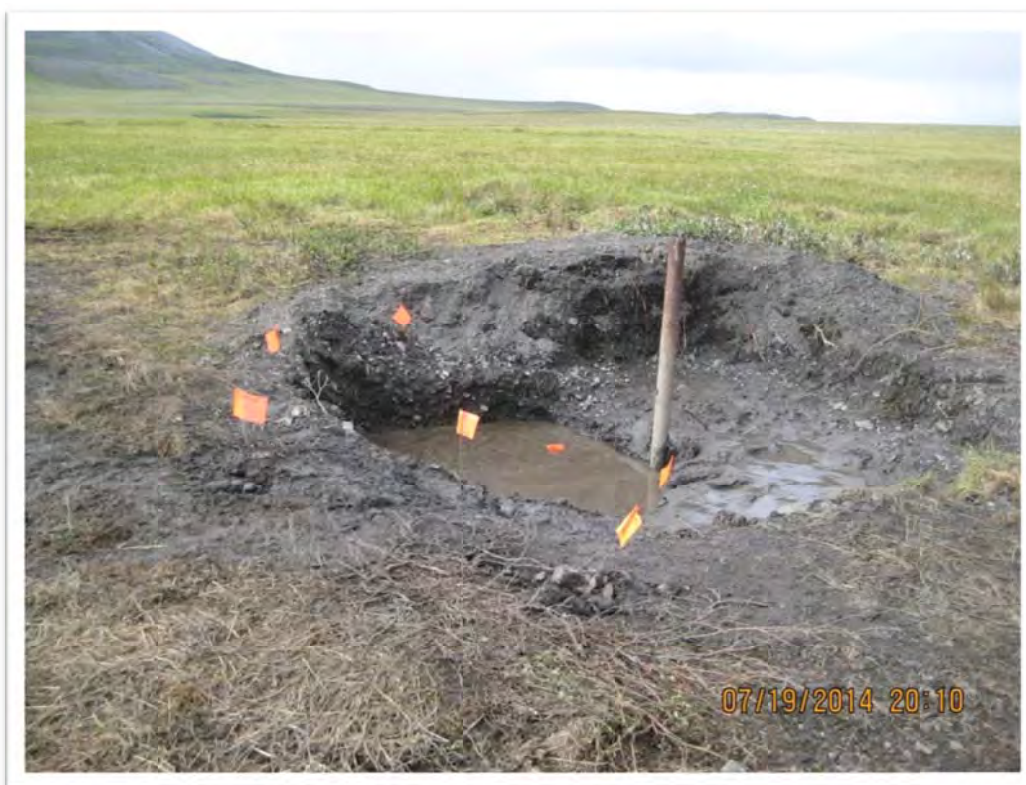
Photograph 18 – Confirmation and footprint sample locations were marked with orange pin flags so they could be surveyed. View to the north.
