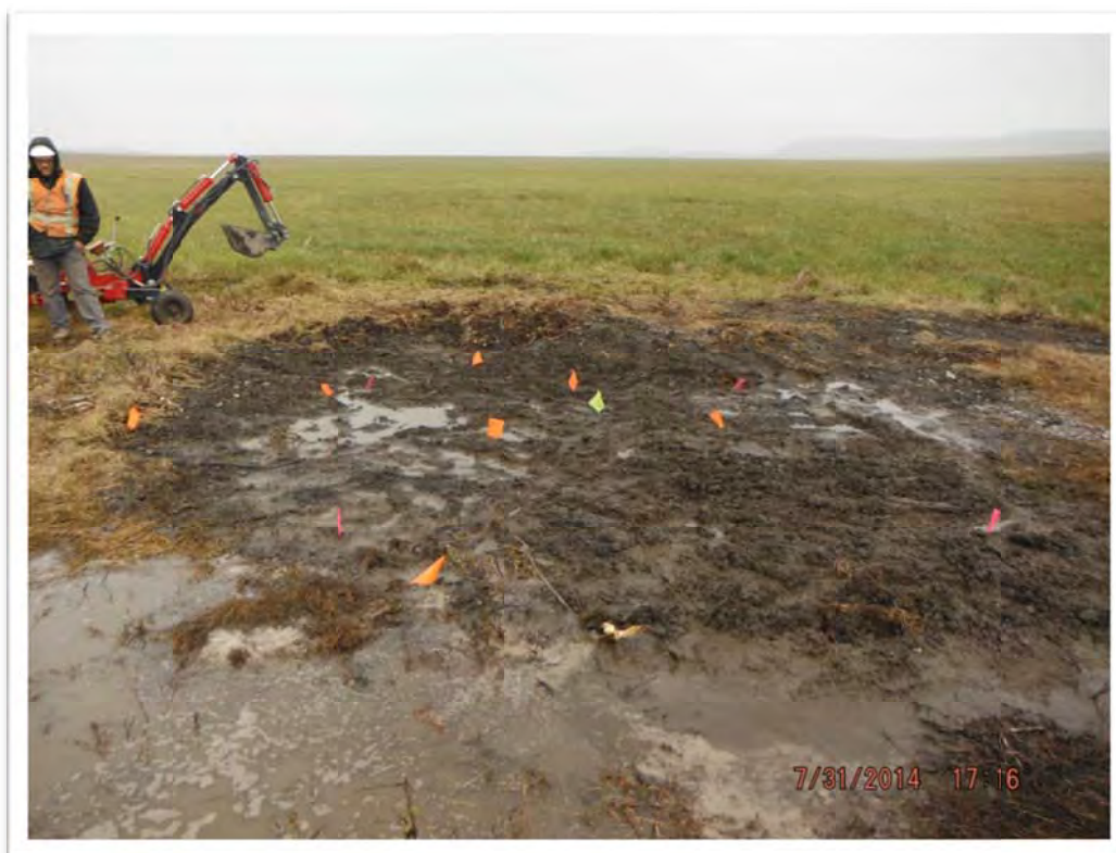
Photograph 19 – View of Test Hole Baker excavation immediately after backfilling and re-contouring. Casing was cut and capped below grade. View to northeast.
