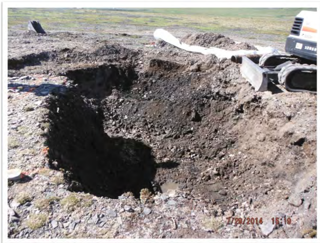
Photograph 45 – Soils closest to the Test Hole X-1 casing appeared to have been previously disturbed. A soil screen, wood debris, gasket and plug were unearthed. View to south.
