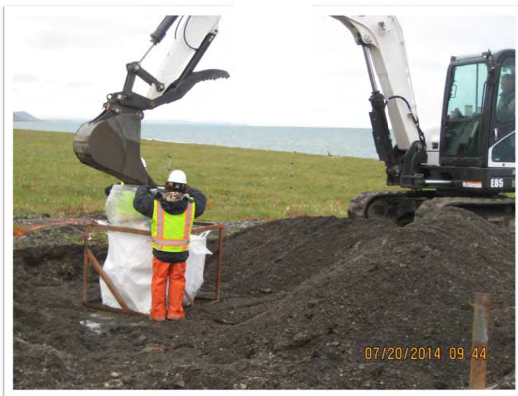
Photograph 23 – POL-contaminated soil was placed in super sacks. View to the southeast.
