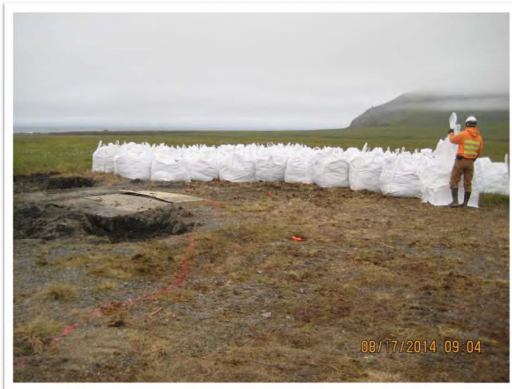
Photograph 36 – Filled super sacks were stockpiled adjacent the Test Hole Dog excavation prior to arrival of additional mud mats. View to the southwest.
