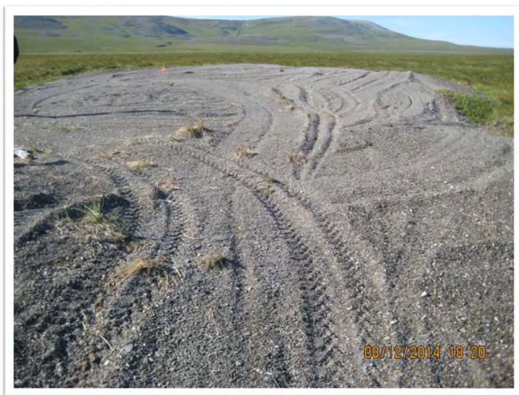
Photograph 13 – Test Hole Able pad was re-contoured following the decommissioning of the casing. Orange pin flag represents the casing location. View to the northwest.
