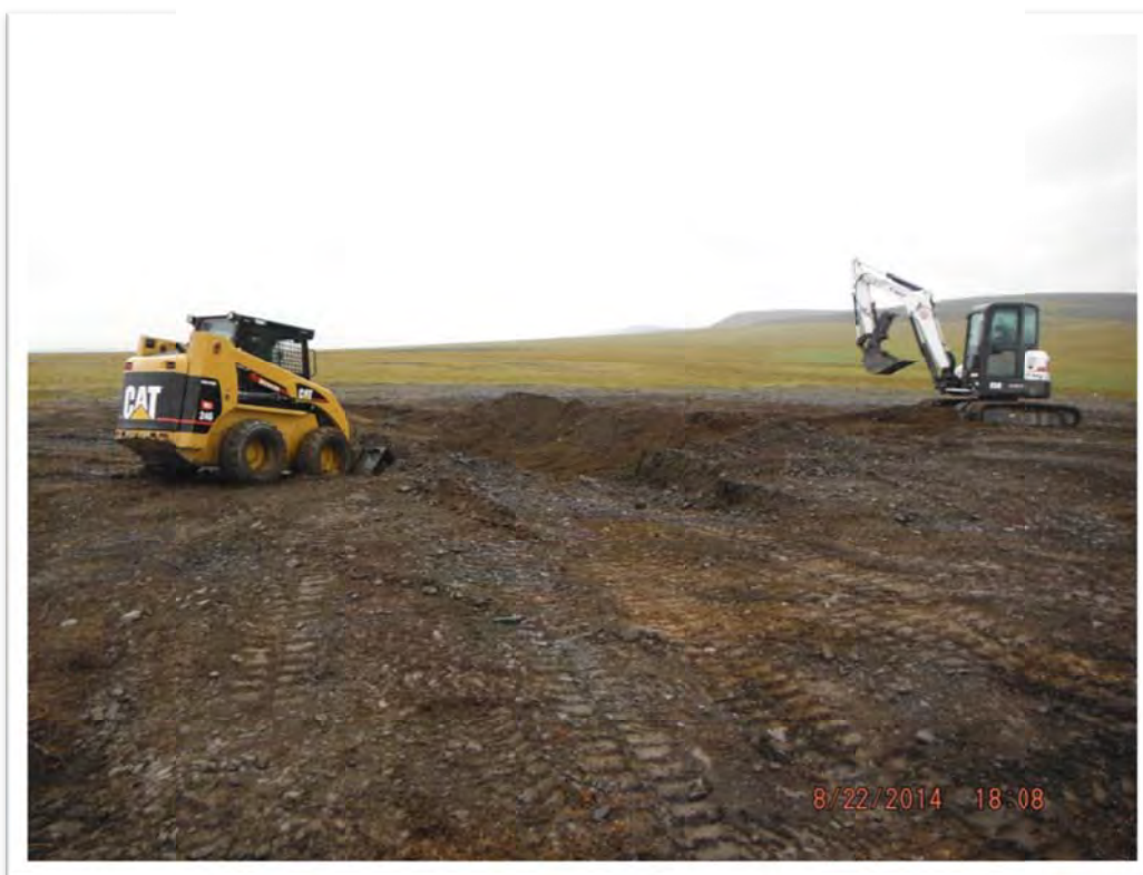
Photograph 51 – Test Hole X-1 was backfilled and contoured to match the existing grade using both excavators and the skid steer and local material. View to northeast.
