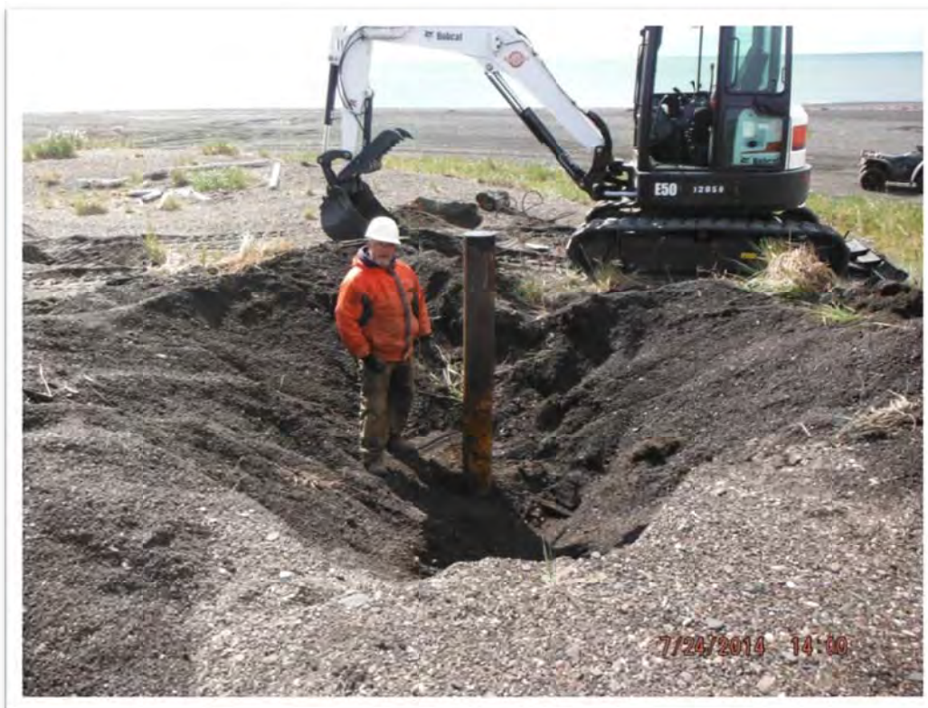
Photograph 9 – The area surrounding Test Hole Able casing was excavated so it could be cut and capped below grade. View to the south.
