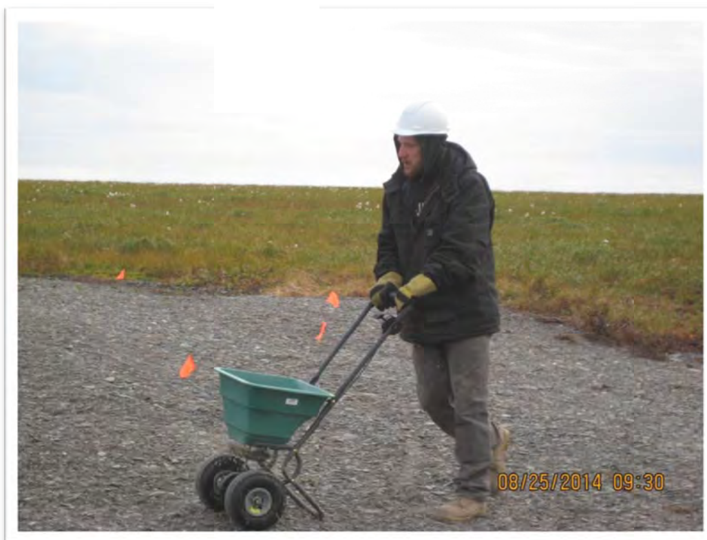
Photograph 31 – Seed and fertilizer were spread on test hole pads following re-contouring. Orange pin flags denote laboratory sample locations with were surveyed on August 27. View to the northeast.
