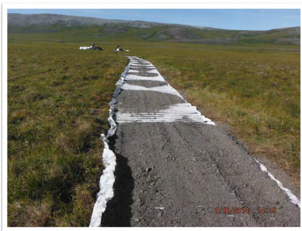
Photograph 34 – Improvements, including the addition of gravel and mud mats, were required to access and remove the filled super sacks from the Test Hole Dog site (site shown in distance). View to the west.
