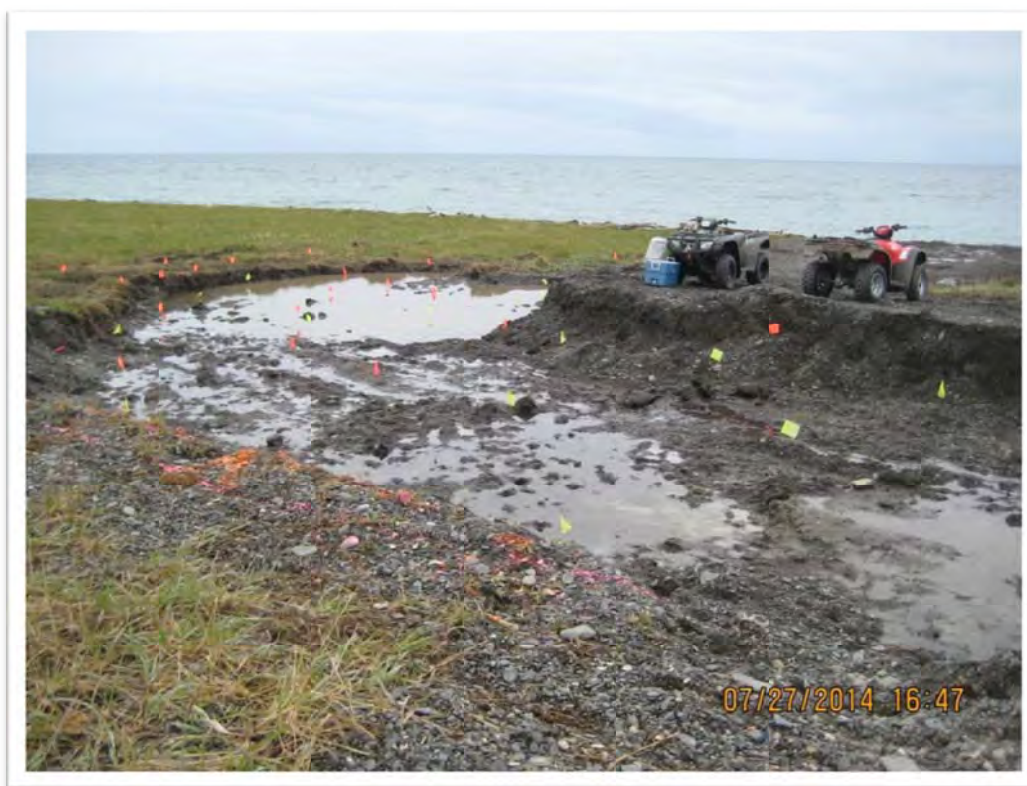
Photograph 30 – Test Hole Charlie excavation looking southeast. Yellow flags represent PID screening locations. Orange flags represent PID screening and laboratory sample locations. Casing is to the right of photograph.
