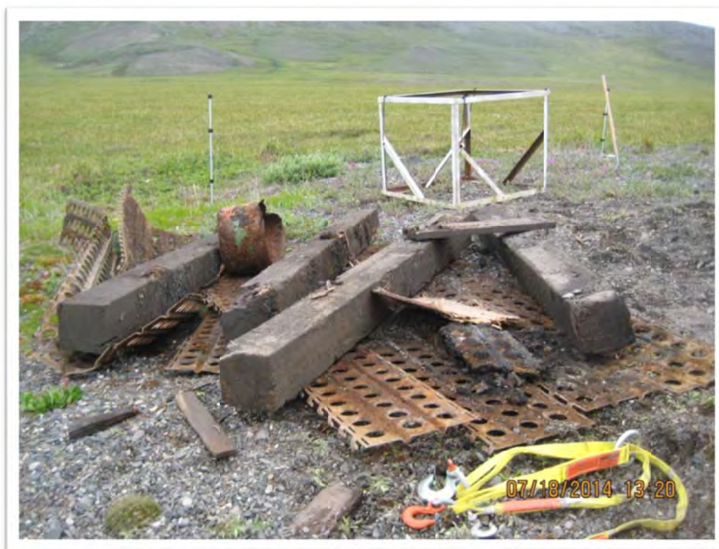
Photograph 24 – View of buried items (overcasing, timbers, and Marsden mats) removed during the Test Hole Charlie excavation. View to the northwest.
