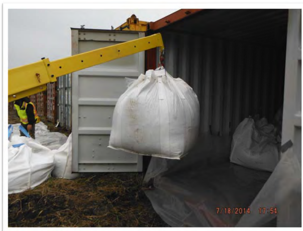
Photograph 56 – Filled super sacks being loaded into the connex shipping containers using an extended boom forklift. Approximately 20 tons of POL-contaminated soil was loaded into each connex.
