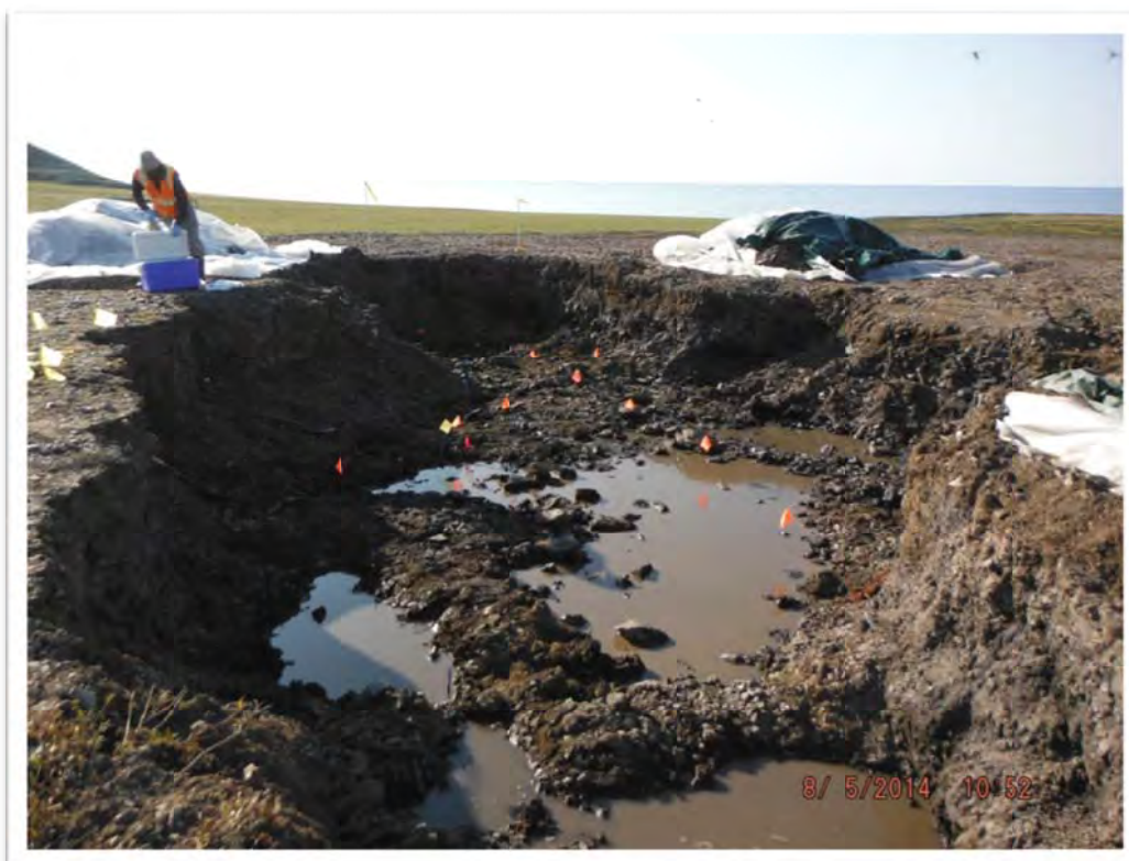
Photograph 49 – Final limits of the Test Hole X-1 excavation. Pin flags mark confirmation sample locations. A total of four stockpiles were constructed around the excavation. View to south.
