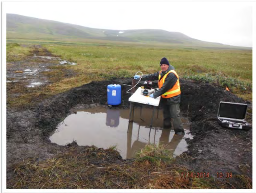
Photograph 16 – Water was pumped from the casing prior to decommissioning. View to the northwest.
