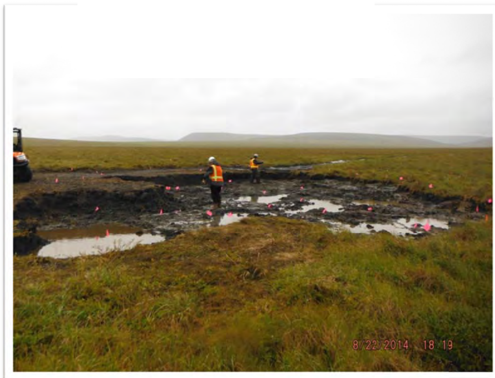
Photograph 40 – Final limits of Test Hole Dog excavation. Pin flags denote laboratory confirmation sample locations to be surveyed. View to the northeast.
