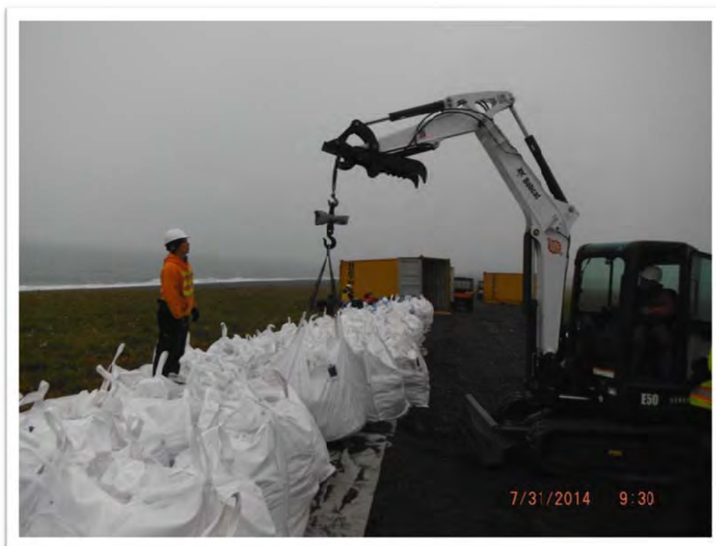
Photograph 54 – Filled super sacks were weighed using a crane scale suspended from an excavator at the staging areas. View to the southwest.
