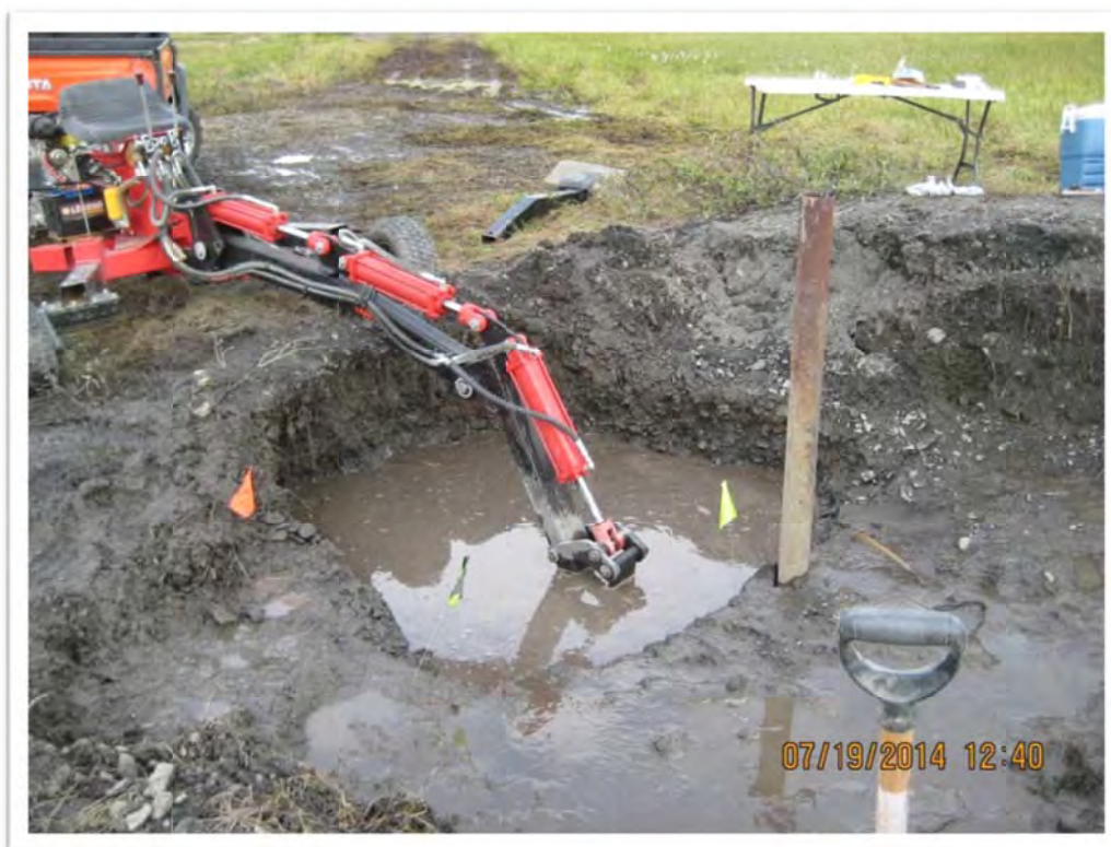
Photograph 17 – The northwest corner of the Test Hole Baker was excavated to a depth of 40 inches. A small, towable backhoe was used due to site access and small excavation size. View to the northwest.
