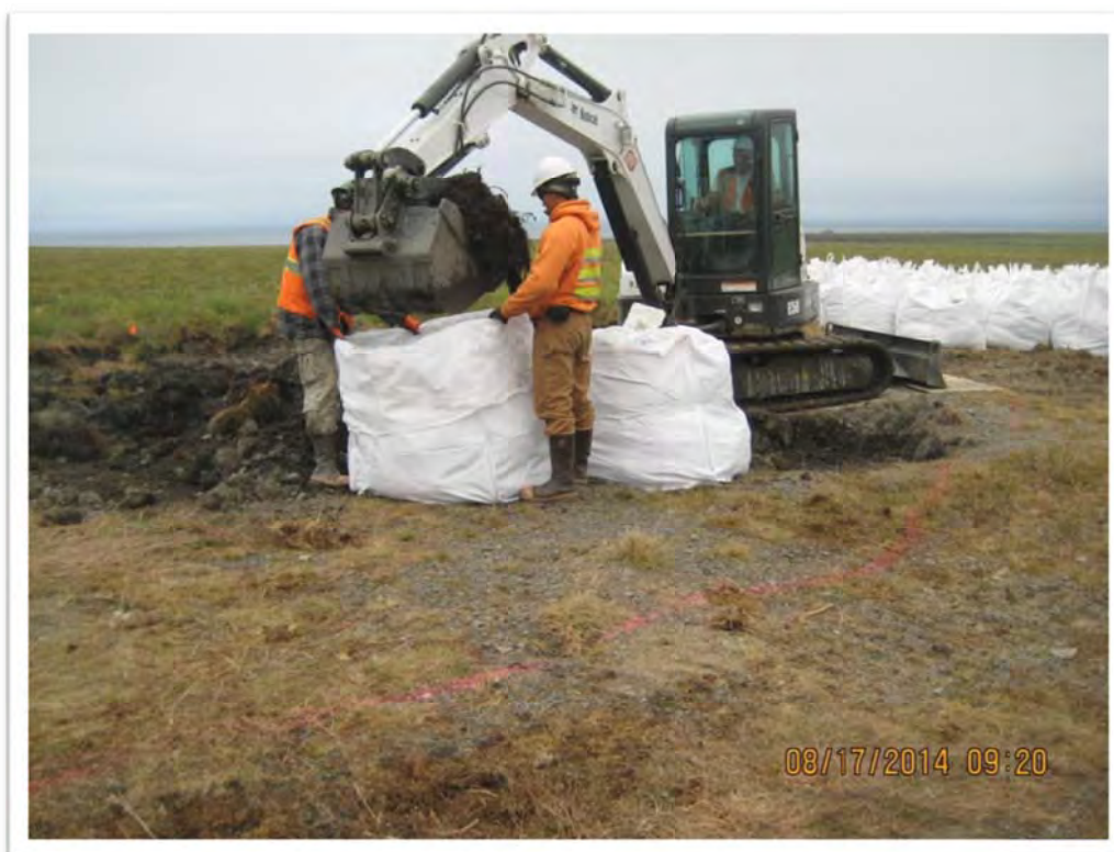
Photograph 35 – Loading super sacks within the Test Hole Dog excavation (see pink spray paint). Note excavator on mats to reduce contact with POL-contaminated soil within excavation. View to the south.
