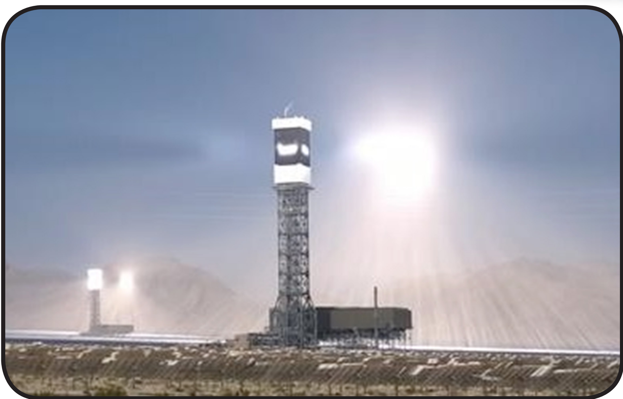
Heliostats in standby mode illuminate regions next to the receiver at the Ivanpah Solar Electric Generating System. New aiming strategies, which minimize the number of heliostats in standby and spread out the aim points, were implemented based on Sandia's analysis to reduce hazards associated with glare and solar flux.
