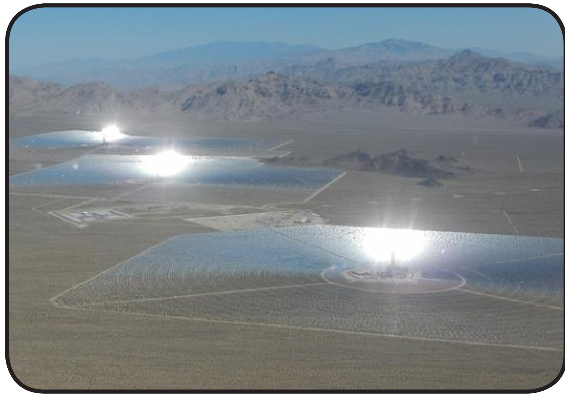
Complaints of glare from pilots flying over the Ivanpah Solar Electric Generating System were evaluated by Sandia and found to be caused by heliostats in standby mode. Sandia worked with NRG and Brightsource Energy to resolve the problem.
