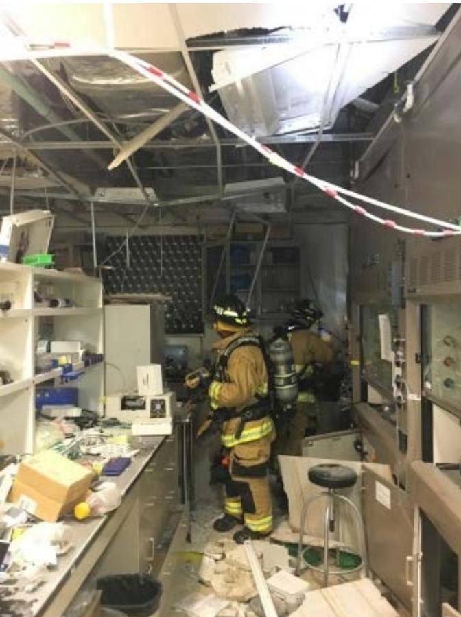
Explosion was due to the detonation of **a large volume of explosive gas mixture** including: Hydrogen, Carbon Dioxide, and Oxygen within the tank.
