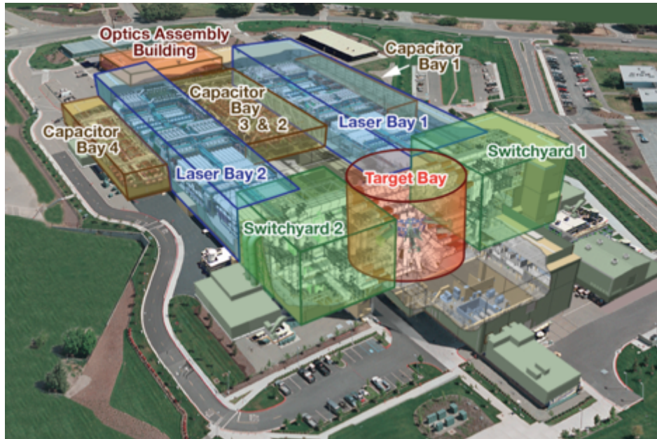
Fig. 5: Top-level optical architecture of the NIF Facility. Spatial-filter telescopes and large 1\omega amplifiers (wavelength of 1.053\text{ }\mu\text{m} ) are most evident in the laser bays. Switchyards house the transport mirrors; capacitor bays store electrical energy for energizing the large amplifiers; light is converted to 0.351\text{ }\mu\text{m} in the target bay, just before entering the target chamber.
