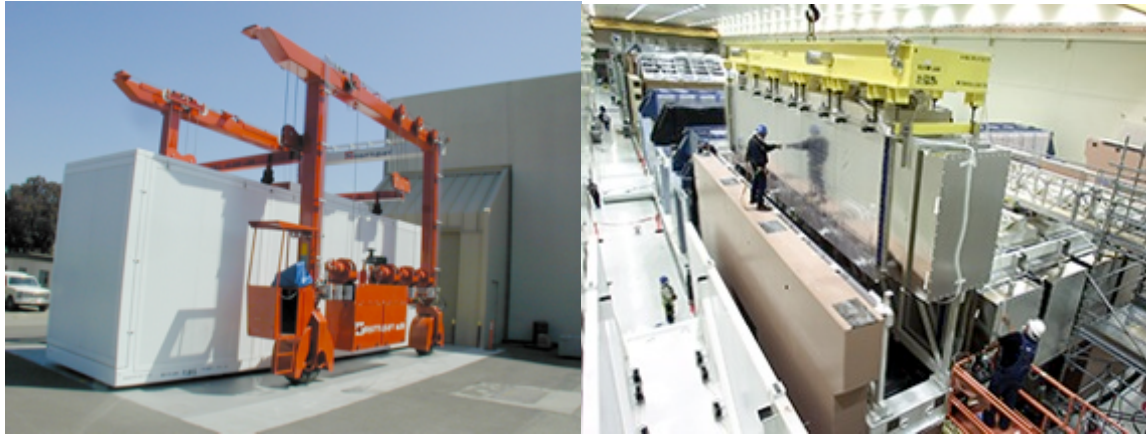
Fig. 53 (a) Transporter delivering an already internally aligned FAU. (b) An FAU being lowered into place in the laser bay.
