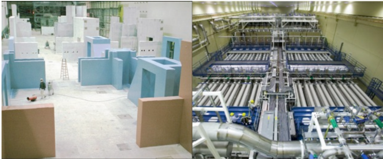
Fig. 10: The Beampath Infrastructure System Exoskeleton of the NIF laser. (a) BIS with the first of its large concrete support structures installed; (b) complete and ready for installation of LRUs.
