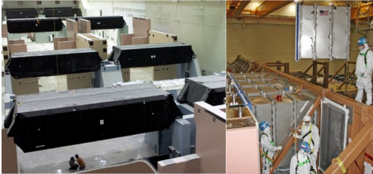
Fig. 11: (a) Spatial filter center and end vessels, triple wrapped and awaiting connection to adjacent BIS hardware (b) Photo taken during installation of a clean bundle-sized beam tube between the LM3s and the Power Amplifiers of that bundle.
