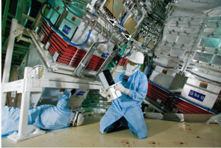
Fig. 89: Installation of the last LRU to go into NIF, (other than those for the final optics) a SIDE camera/shutter assembly for Quad 45B. This SIDE assembly will be placed into the beam enclosure just above the floor on which one of the installers is kneeling, about 3 m upstream from the location of the TCVWs (indicated by the arrows, black with white surrounds).
