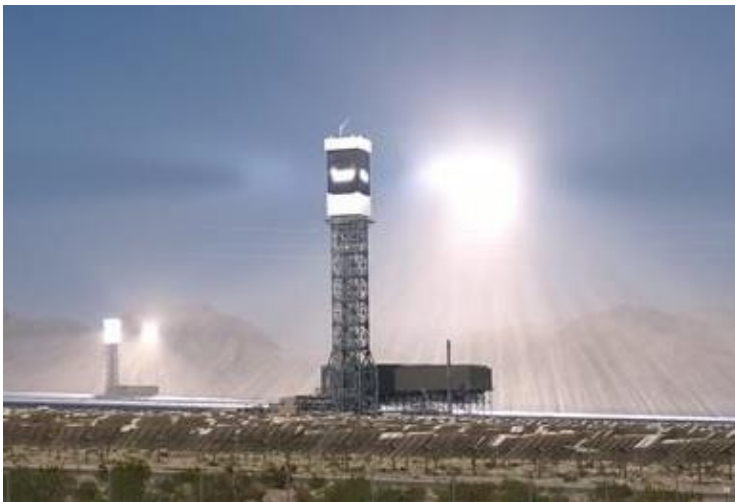
Photo and model of high-flux regions causing solar glare and avian hazards at Ivanpah Solar Electric Generating System
