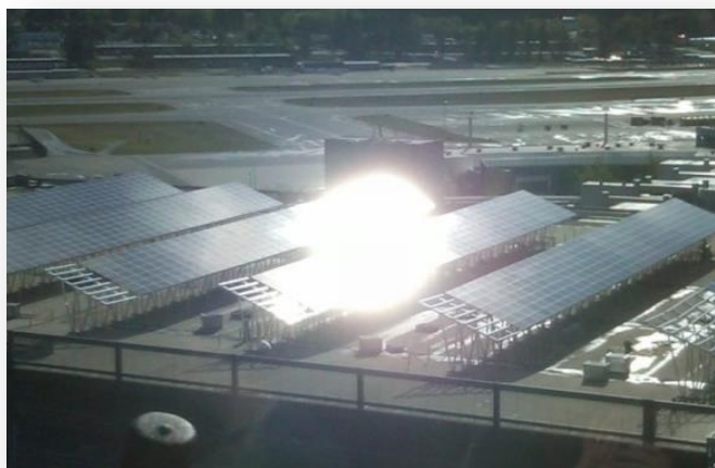
Glare observed from control tower at Manchester-Boston Regional Airport ($3.5M construction; $2M to reconfigure)
