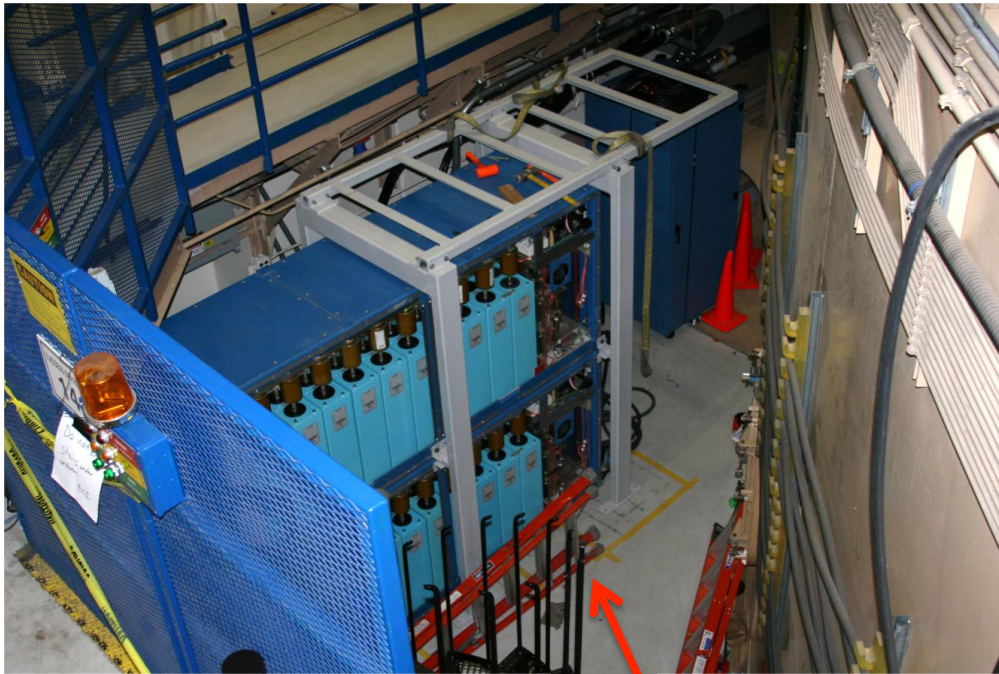
Photo of capacitor bank w/o covers; with covers →
