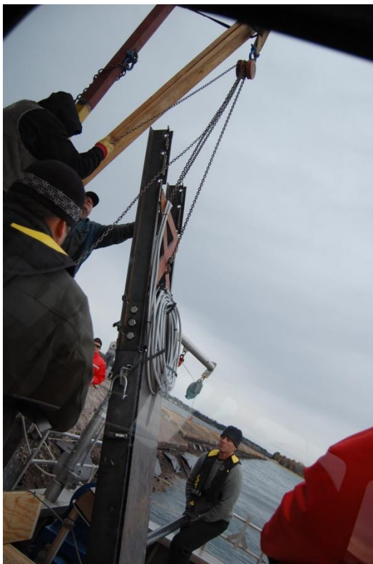
Figure 5.3.(a) Installation of Ice Force Measuring System's pressure plate
