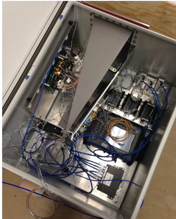
Figure 6.5 WiBAR completed assembly
