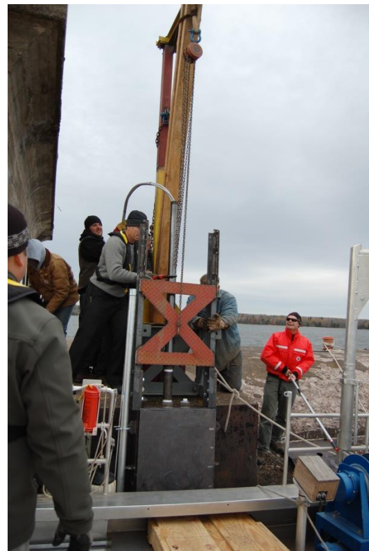
Figure 5.3.(a) Installation of Ice Force Measuring System's pressure plate
