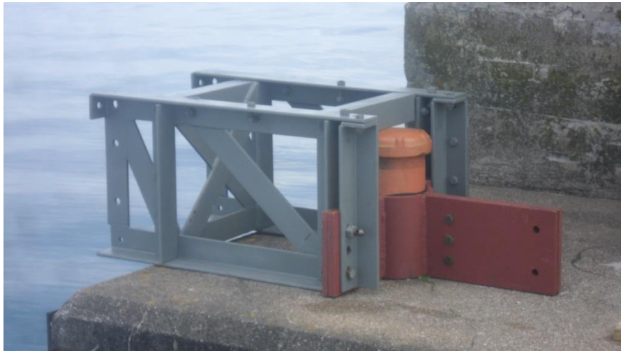
Figure 5.2 Bollard collar and deck frame after installation
