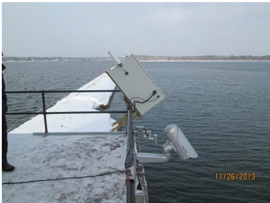
Figure 7.2. Photo showing right stereo camera in foreground, WiBAR system (center), and IFMS camera below WiBAR.
