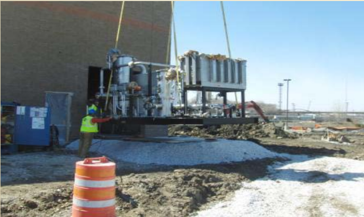
Unloading and placing dryer skid.
