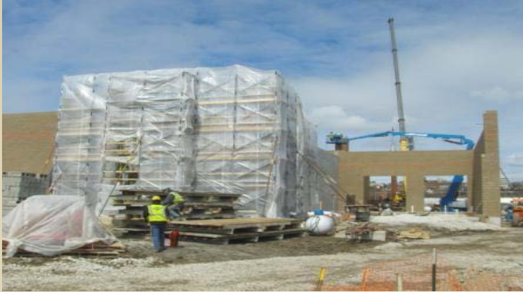
Masonry at Membrane Room
