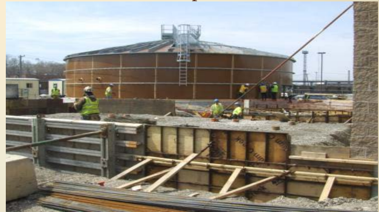
Forming of exterior tank farm slab.
