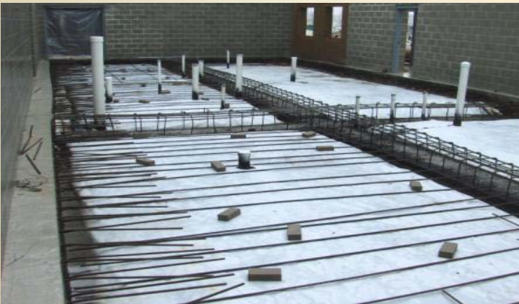
Prepping Maintenance Room floor to pour, methane protection in place.
