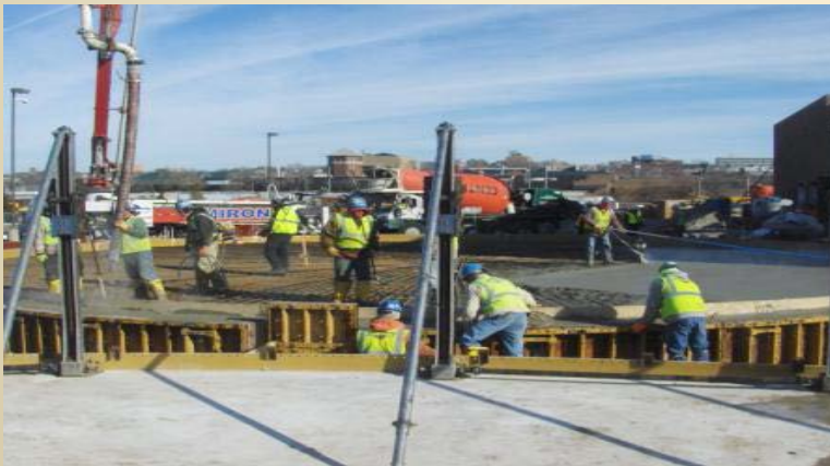
Pouring and Finishing Reactor 1 Slab
