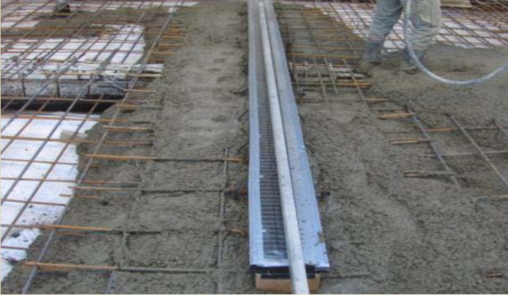
Pouring the centrifuge floor.
