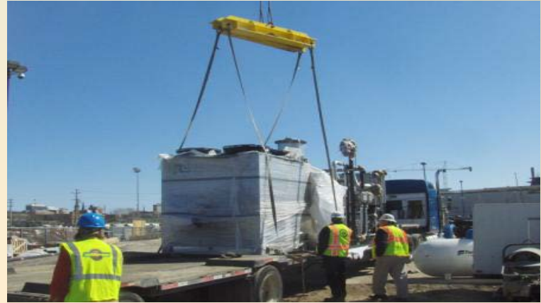
Unloading and placing dryer skid.
