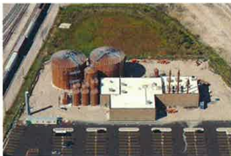
The 2-megawatt (MW) FCPC Renewable Generation facility is located near the Potawatomi Bingo Casino on tribal land in the Menomonee Valley region of Milwaukee, Wis. Miron Construction Co. Inc.
