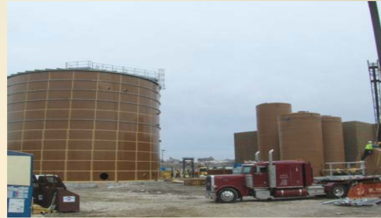
Setting feedstock tanks.
