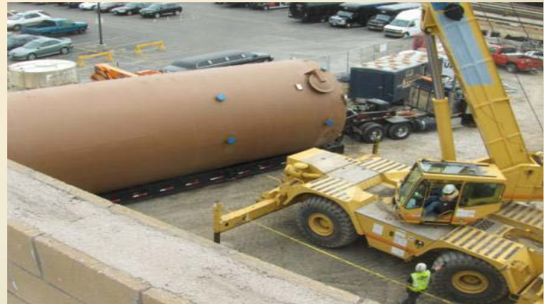
Offloading feedstock tanks.
