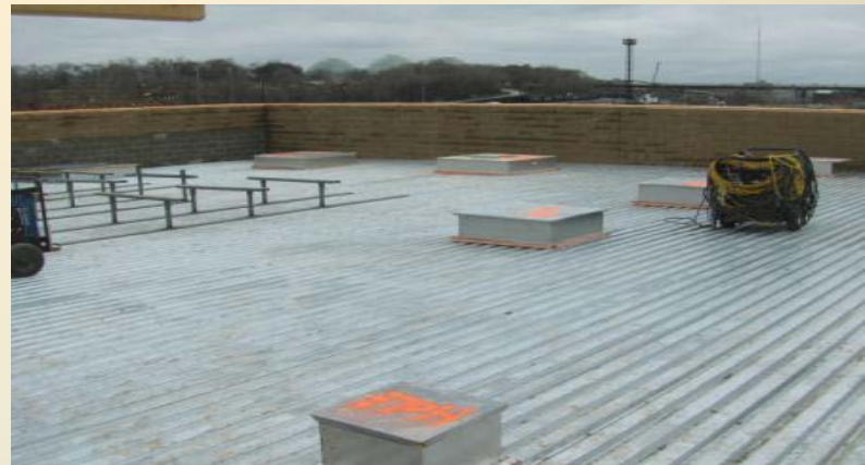
Deck and equipment supports in place, commence roofing over Engine Room.
