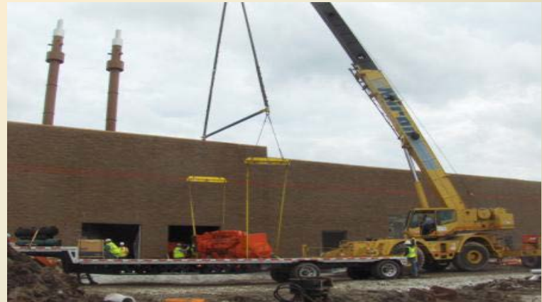
Unload and set engines.
