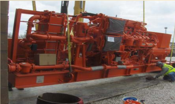
Unload and set engines.
