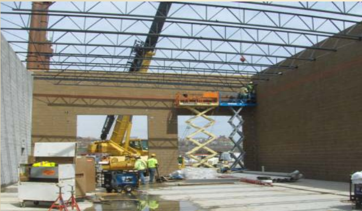
Set bar joist in truck unloading.
