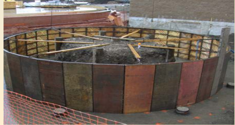
Form equalization tank walls.
