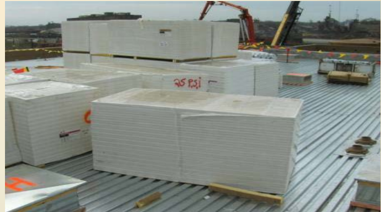
Unloading materials for remaining roof.
