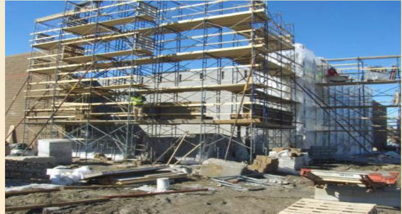
Masonry at Demising Wall
