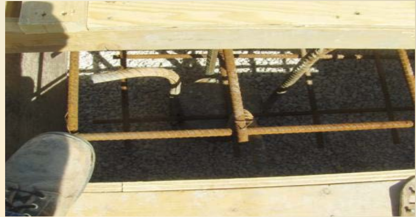
Flare pad forming and reinforcement before pour.
