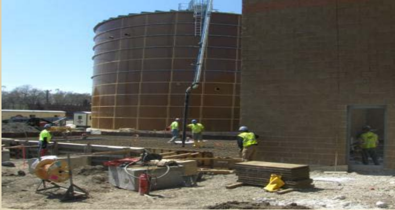
Form and pour exterior tank slab. Note the tank in the background growth.
