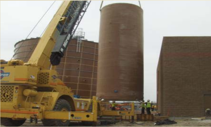
Setting feedstock tanks.
