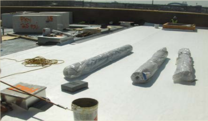
Roof over Engine Room under way.
