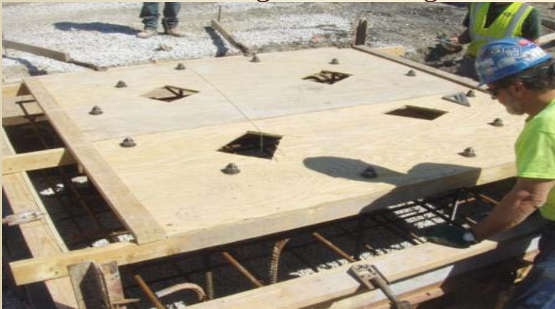
Flare pad before pour, anchor bolt pattern checked.
