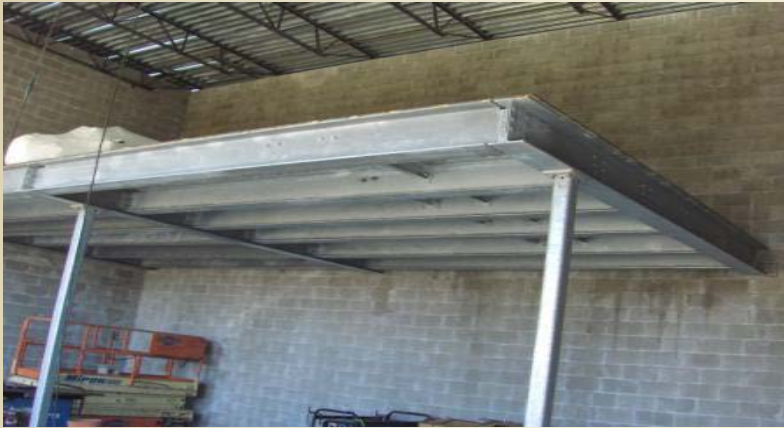
Centrifuge platform erected, waiting for Centrifuge and railings.
