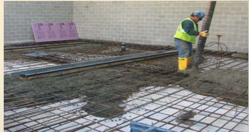
Pouring the centrifuge floor.
