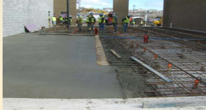
Pouring truck unloading floor.
