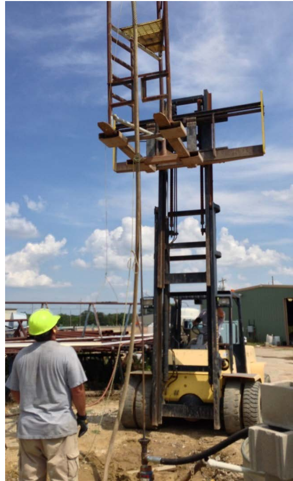
Figure 35b. Jointed Pipe Rig w/ Wellhead
