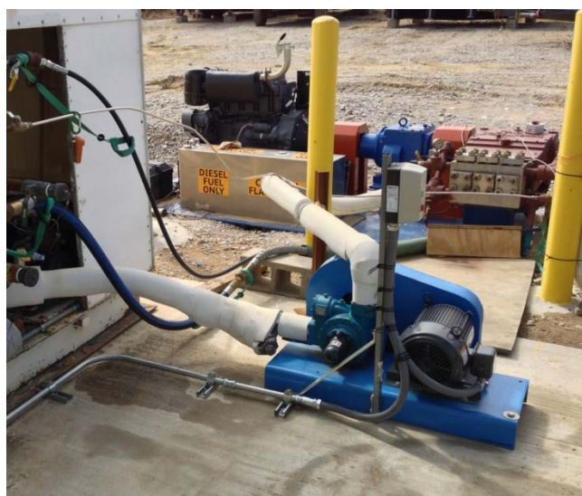
Figure 26. CO 2 Charge Pump installed April 2013
