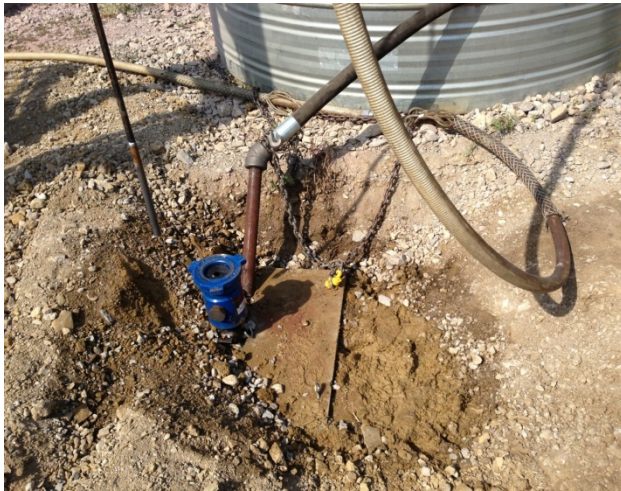
Figure 34. Wellhead & Return Tank for Vertical Drilling
