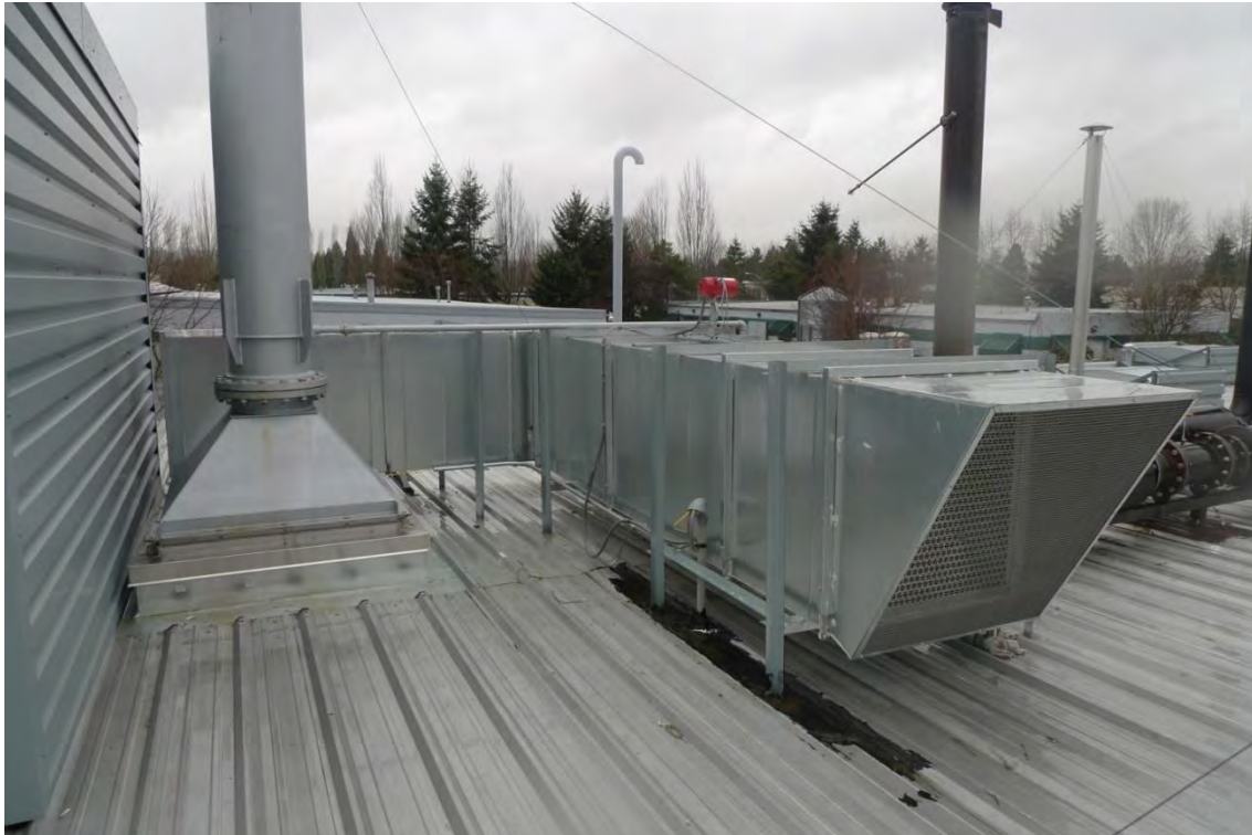
Figure 12.6 - Engine inlet duct (square duct on right).
