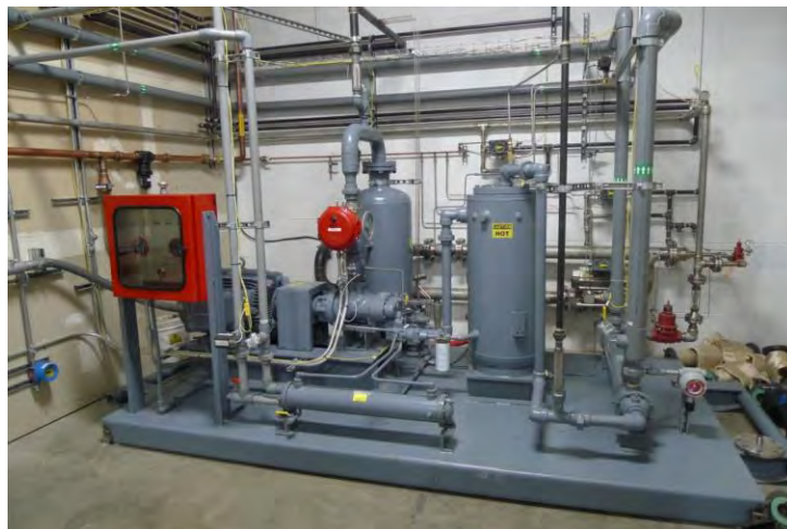
Figure 12.9 - ISCE natural gas supply skid.
