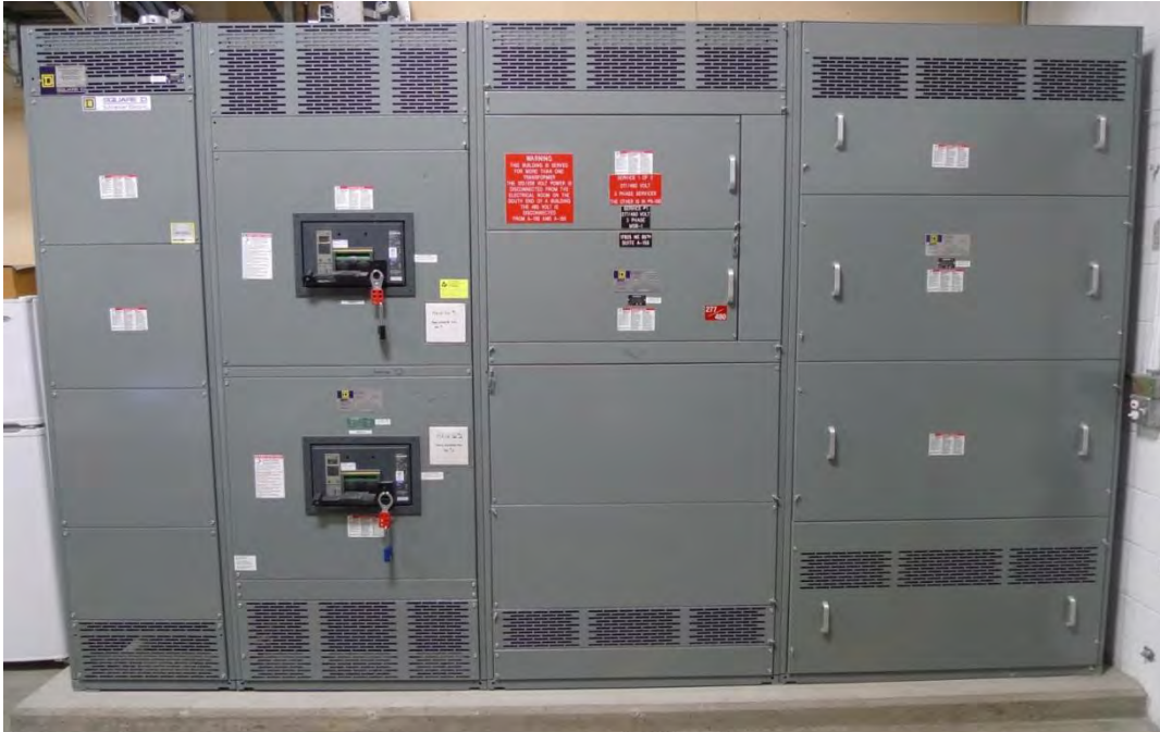
Figure 12.2 - MCC used for 1.5 MW motor.
