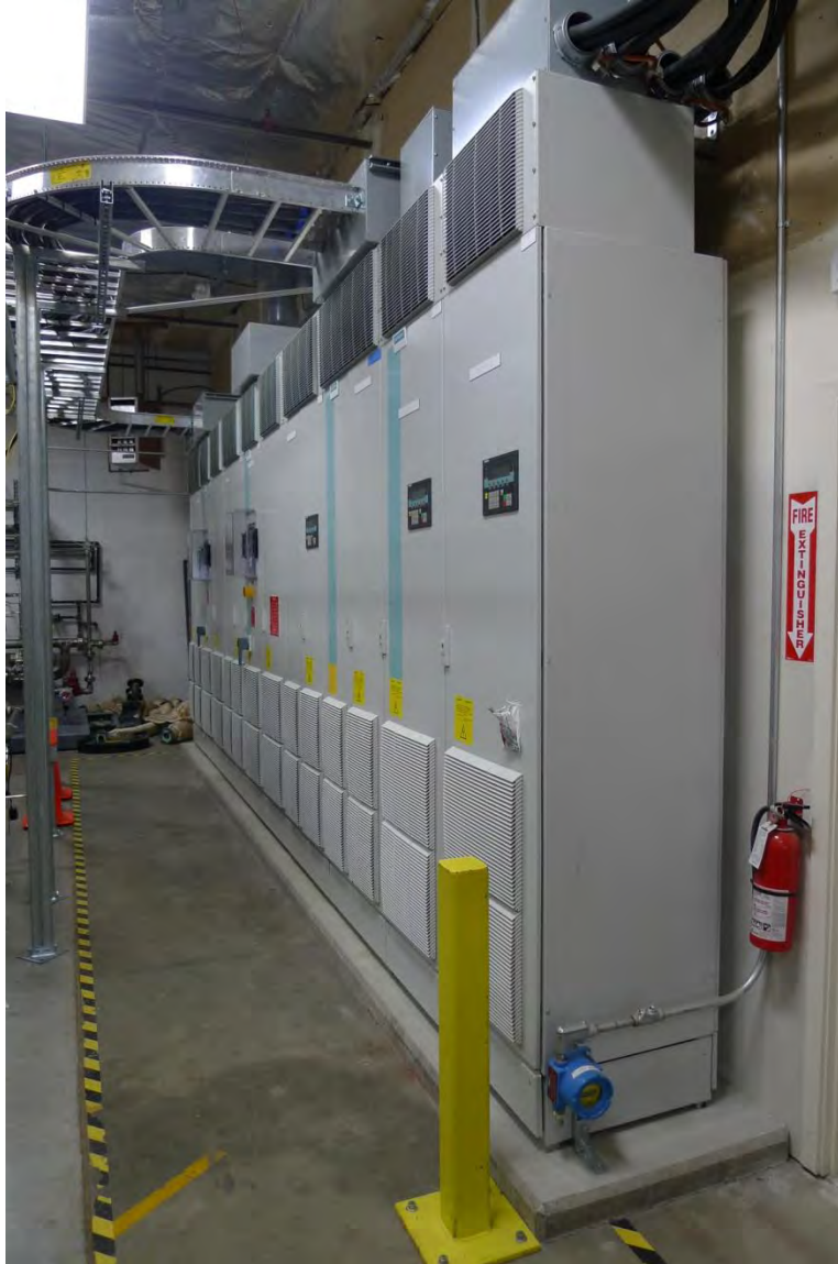
Figure 12.4 - 1.5 MW Variable Frequency Drive (VFD).
