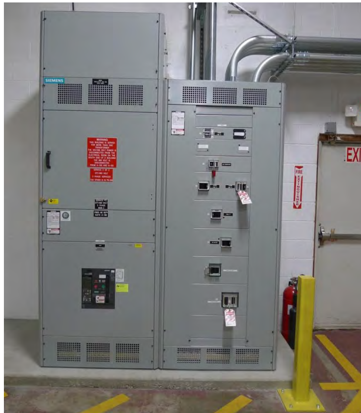
Figure 12.3 - MCC for facility supporting machinery.
