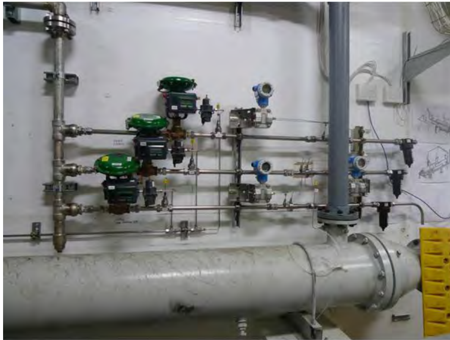
Figure 11.36 - Nozzle cooling air control valves and flow meters installed in Redmond test lab.
