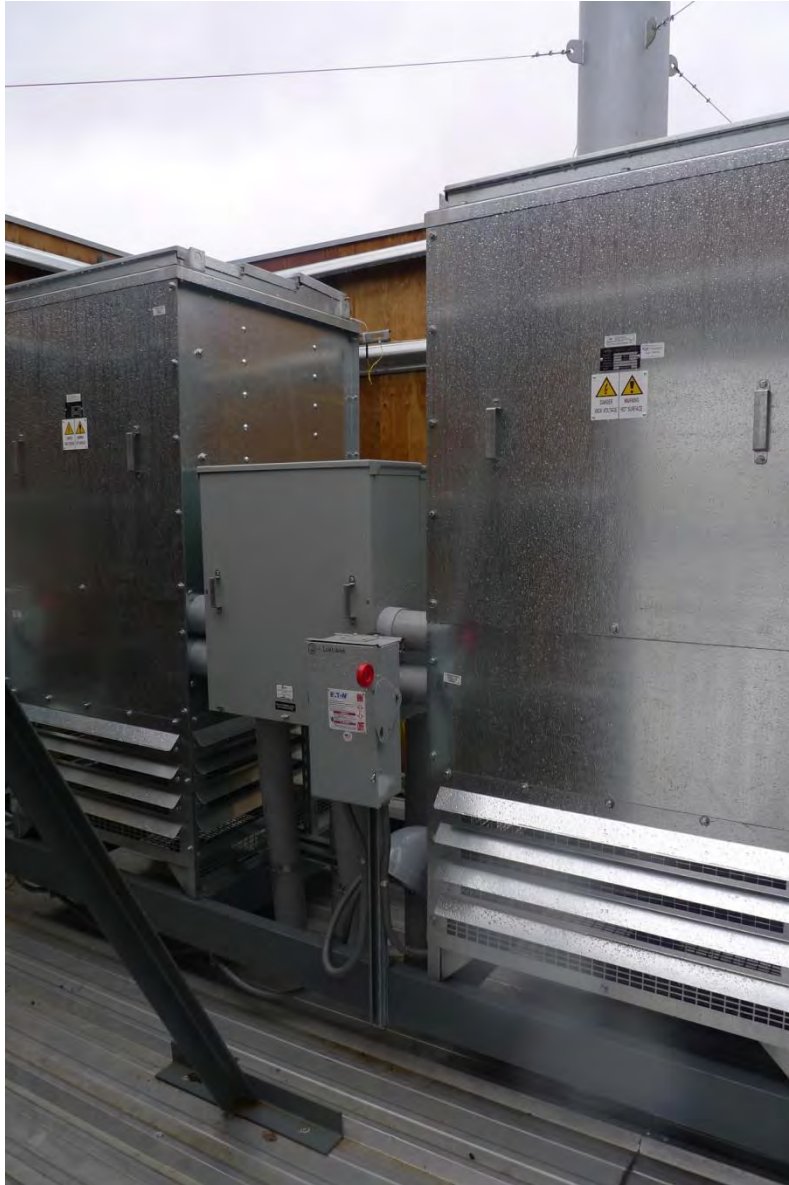
Figure 12.5 - Photograph of roof-mounted engine braking resistors.
