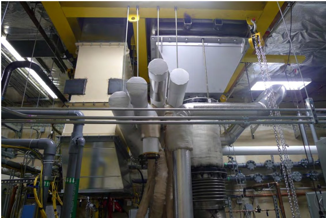
Figure 12.7 - Engine inlet silencer (left) and exhaust silencer (right).
