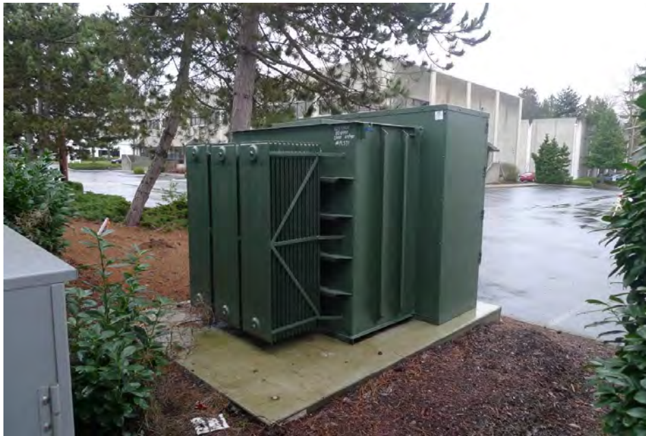
Figure 12.1 - 2500 kVA transformer for ISCE test facility.
