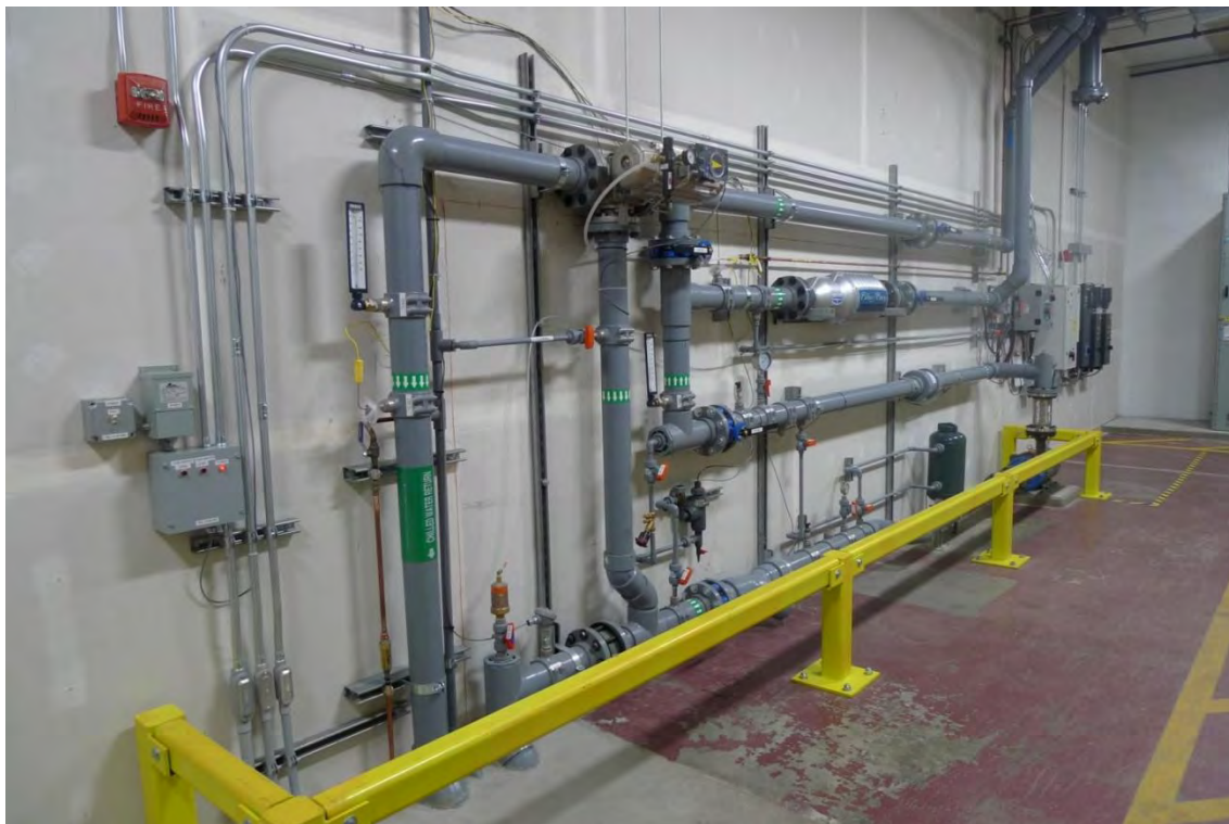
Figure 12.12 - Facility water cooling system plumbing, pumps, and cleaning systems.
