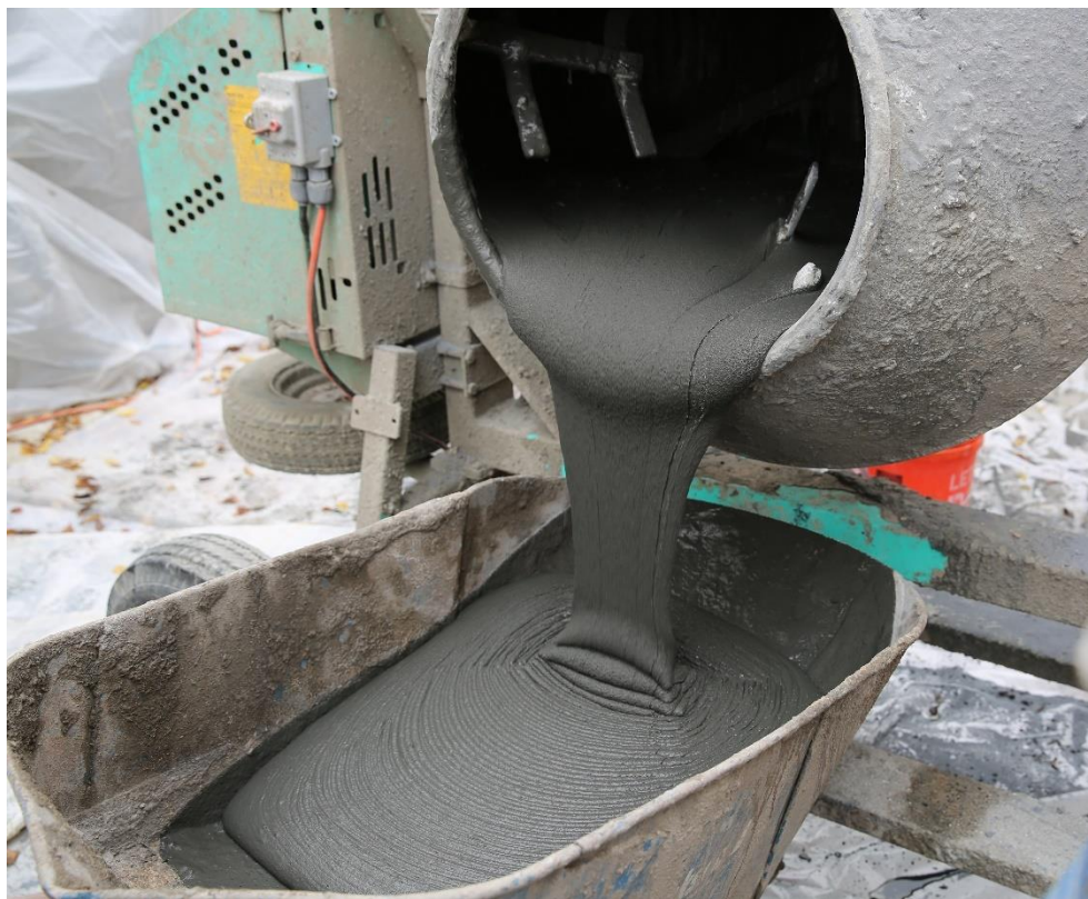
Figure 29. Completion of mixing
