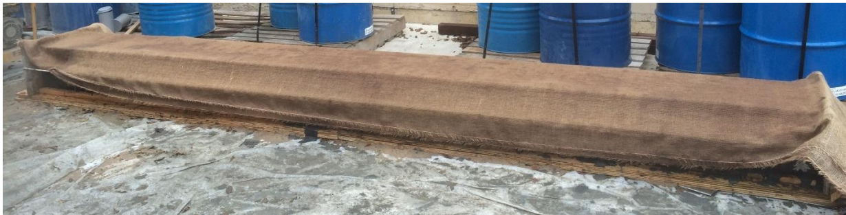
Figure 140. Curing arrangement for S-UHPC beams
