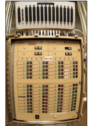
Z's water drain/fill control system In place since 1985.
