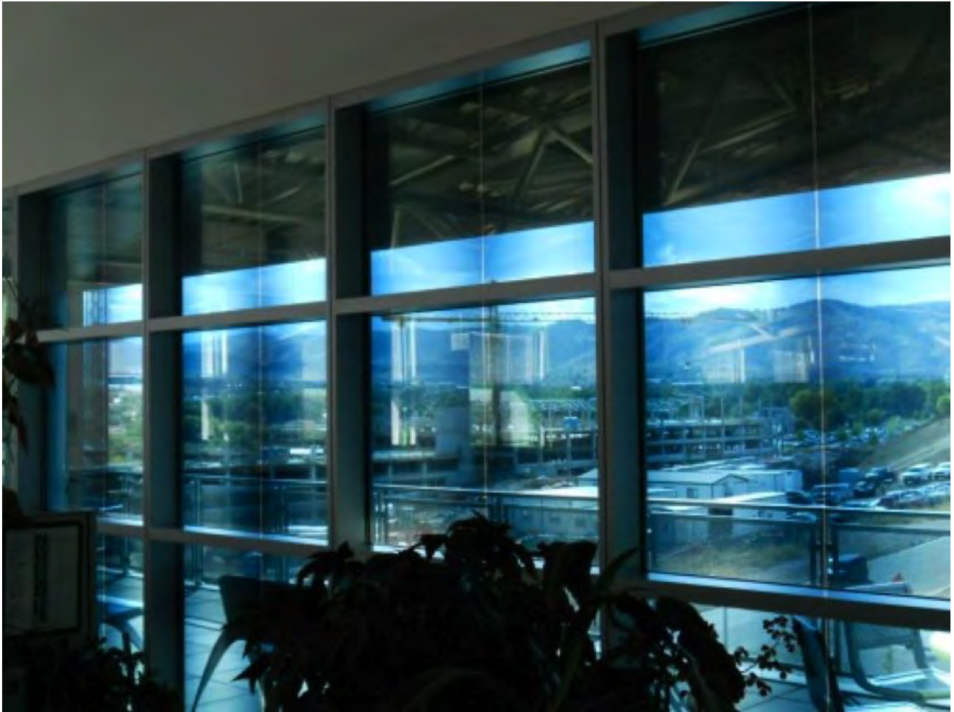
Figure 32: Photograph of the electrochromic window a few minutes after starting to switch. We were unable to obtain images of the windows switching at the Denver Federal Center, but images taken at the National Renewable Energy Laboratory's Research Support Facility [20] illustrate the variation in coloration while switching.
