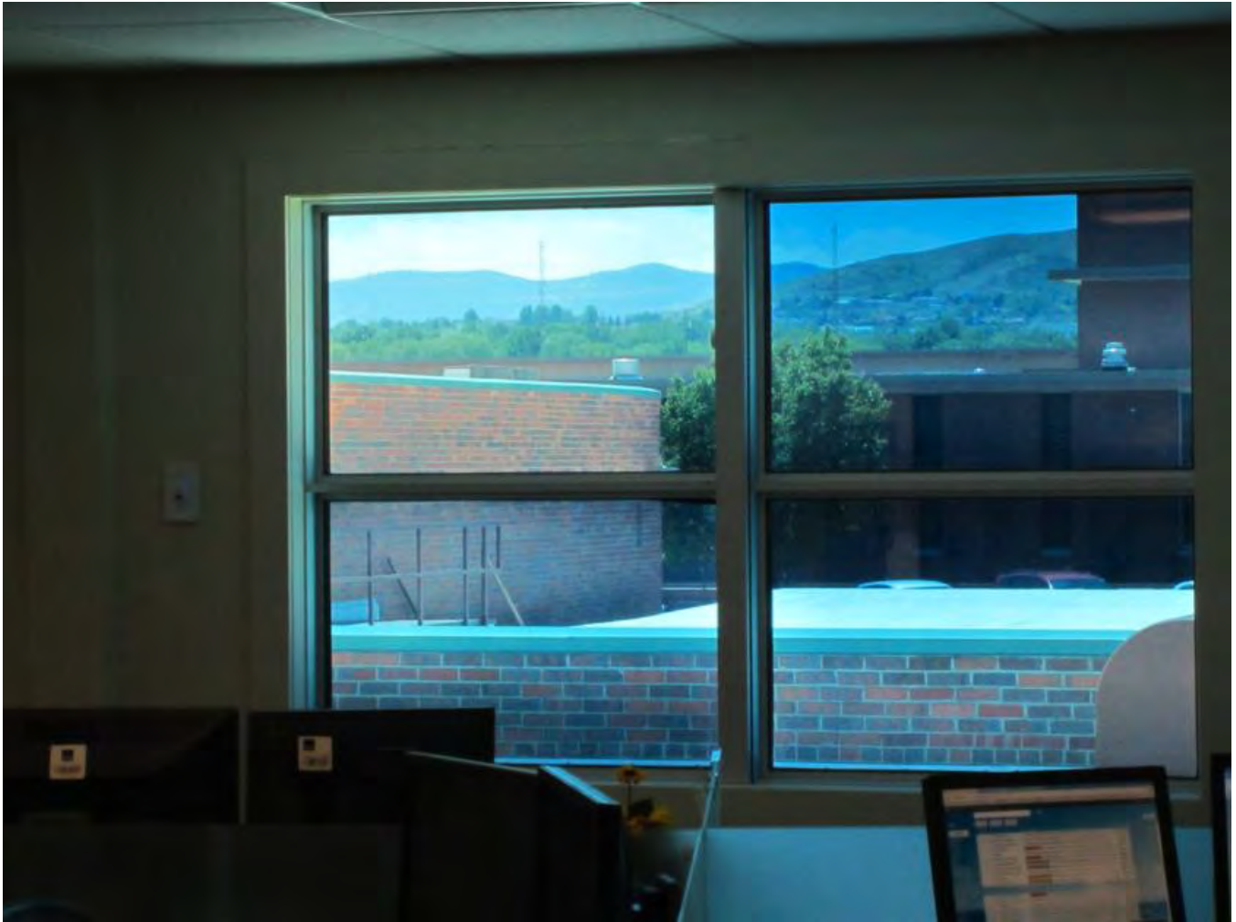
Figure 31: Photograph of an electrochromic window in the perimeter zone during Phase II illustrating the slight differences in tint level between adjacent window panes.
