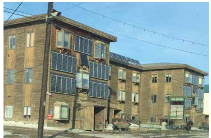
Solar panels are positioned to capture the low angle of the sun in Noatak (left) and Nome.
