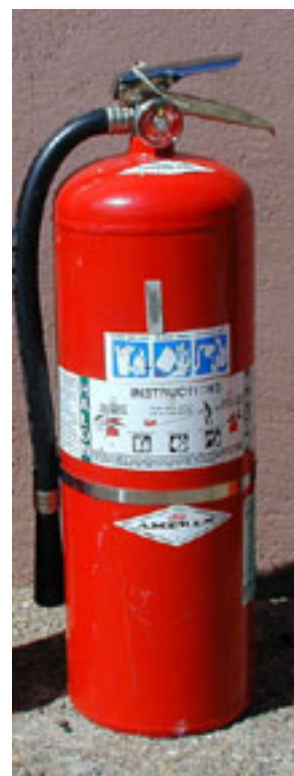
A halon fire extinguisher
