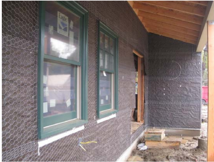
Figure 15 Left : existing, cracked stucco was removed and house was re-clad with a continuous weather resistive barrier beneath the new stucco. Right : Whole-house fan used for nighttime ventilation cooling, insulated and self-sealing when not operating.
