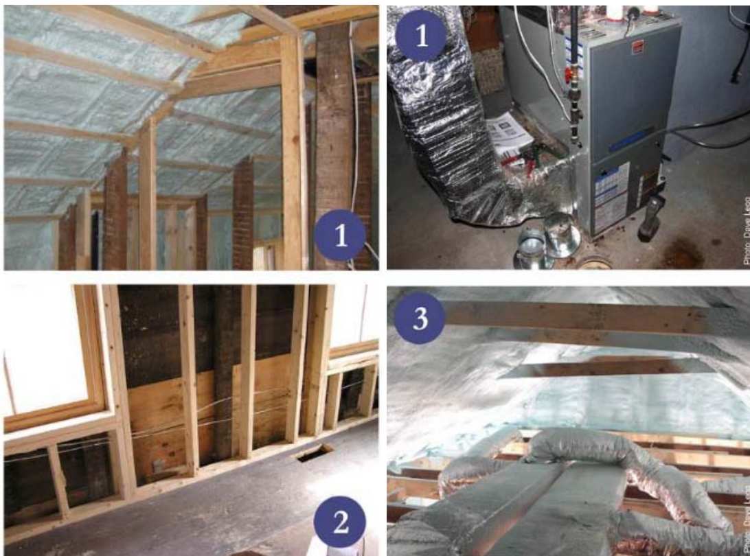
Figure 7 Images from Belchertown DER (clockwise from top left), including sealed and insulated attic, high efficiency forced air gas furnace, new stud wall built to interior of old structure, and HVAC ducting insulated and in conditioned space. Images courtesy of the Building Science Corporation.
