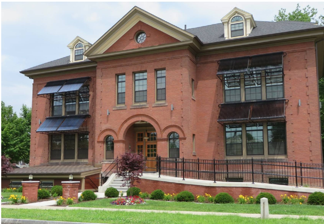
Figure 3. Evacuated-tube solar collectors mounted as awnings over south-facing windows
