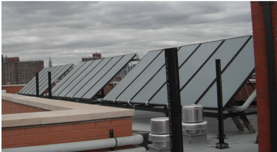
Figure 2. The 960 ft 2 of solar collectors occupy most of the available, unshaded roof area on this six-story multifamily building.
