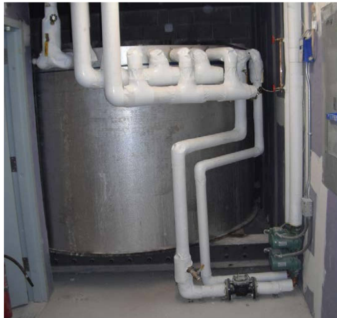
Figure 1. This 1,500-gallon solar storage tank served to preheat water for 59 apartments.
