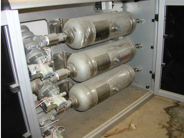
Fig. 3. Inside of the accumulator cabinet. By moving critical parts out from under the bridge, maintenance is much more easily managed.
