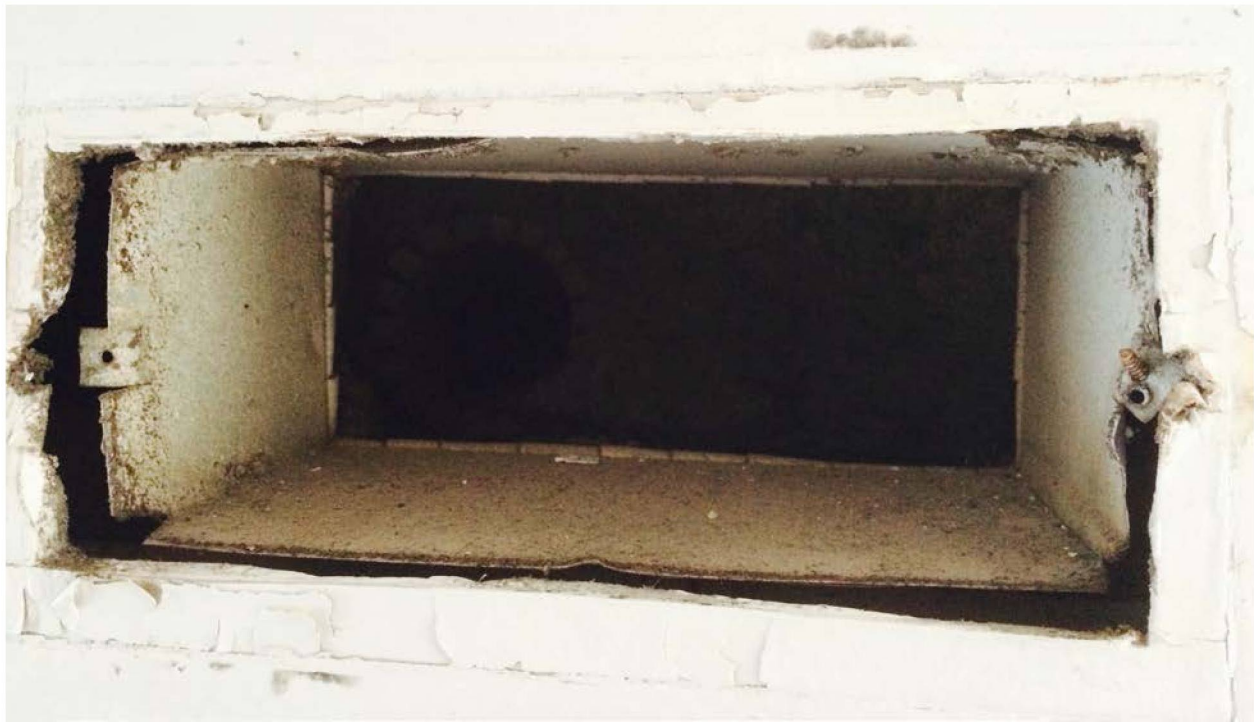
Figure 6. Duct boot not sealed to drywall
